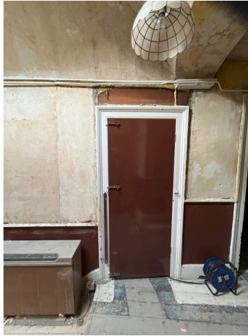
Block (to stair well to 2 nd floor)
