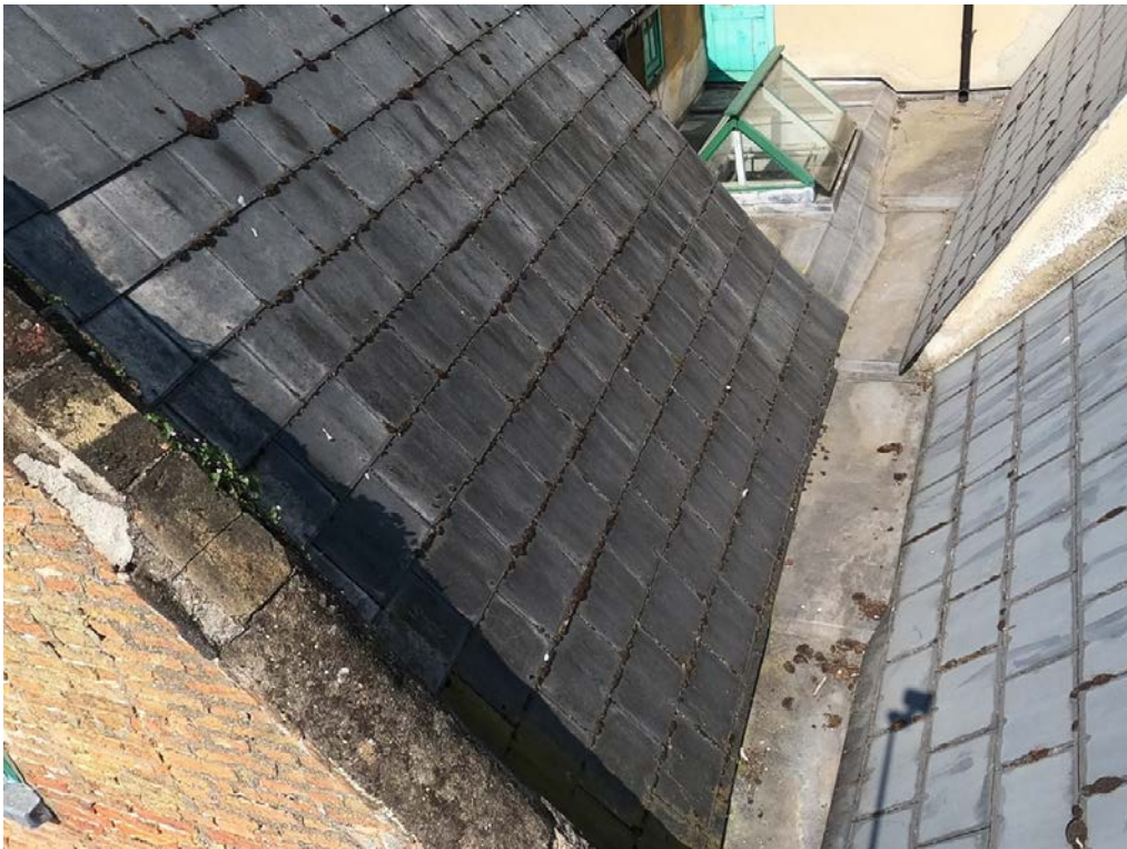
Fig 9. Flat roof area to rear elevation.
