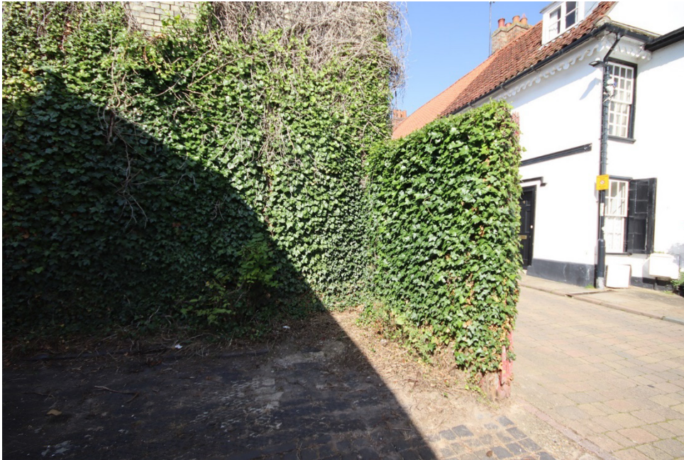
Fig 41 Rear wall to be taken down to allow access.
