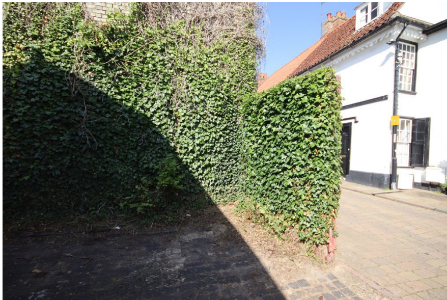
Wall adjacent to Palace Street to be removed.
