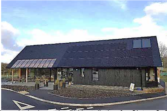
Award winning solar PV installation for Cletwr Café community project, Mid-Wales, 2017
