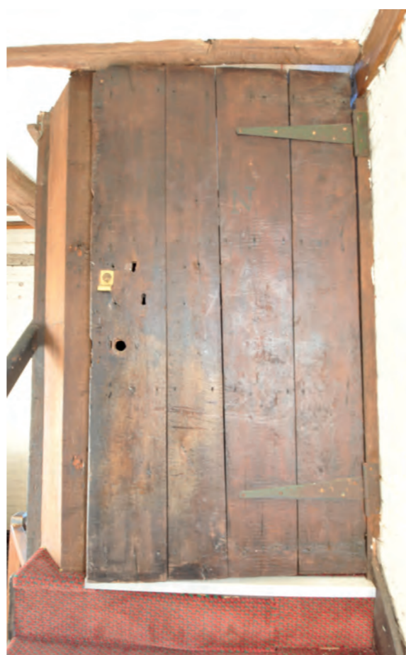
Arch interior of ground floor entrance door - the arch is a secondary insertion cut through a original window opening, the infill of the arch is again later than the arch
