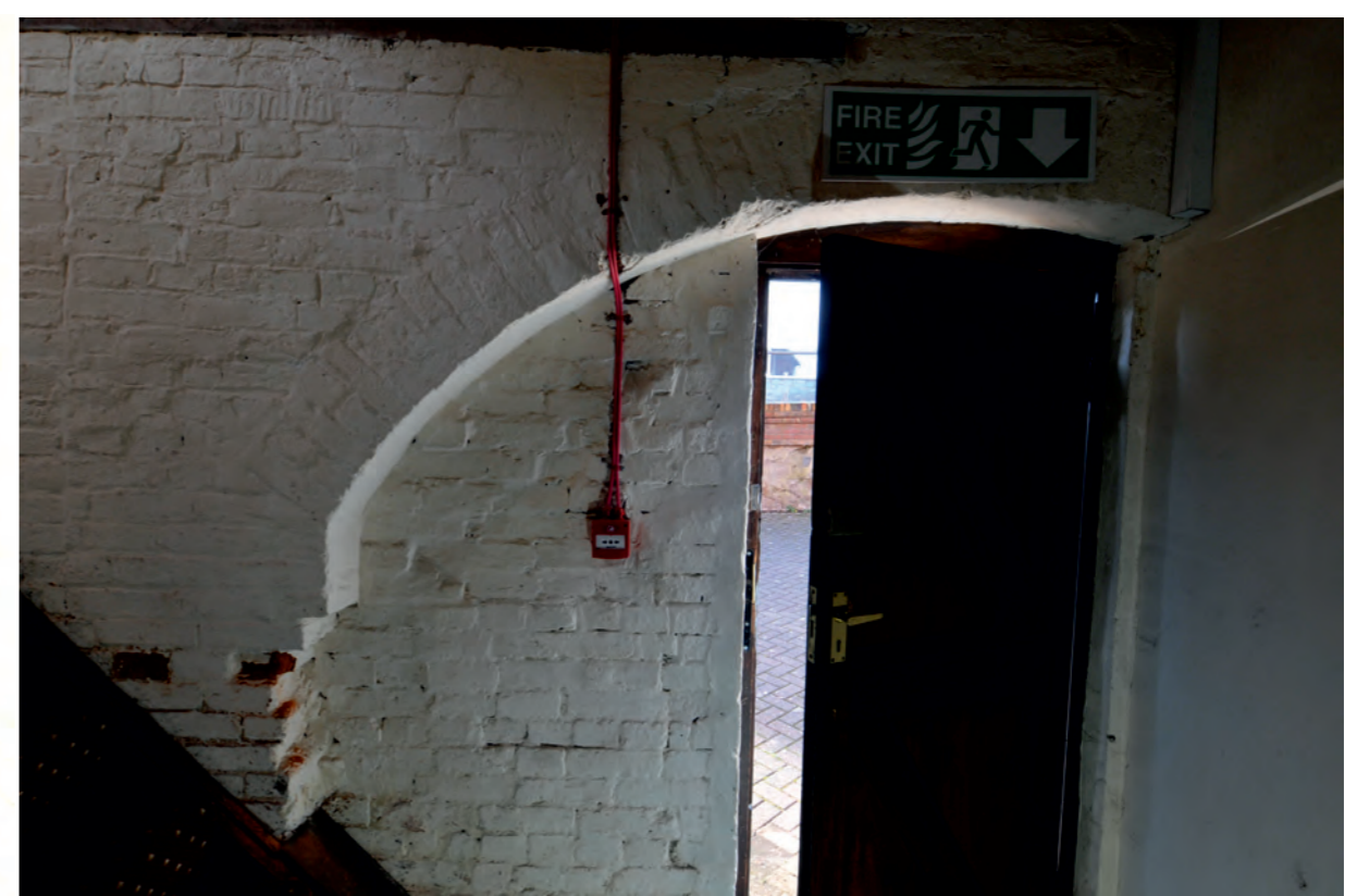
Arch interior of ground floor entrance door - the arch is a secondary insertion cut through a original window opening, the infill of the arch is again later than the arch
