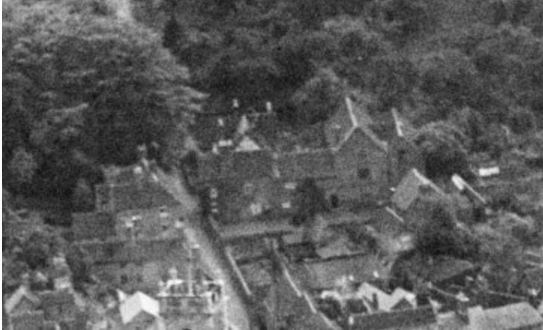
1930s view of warehouse complex from the east
