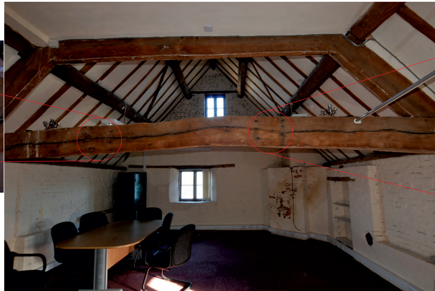
Truss 3 view facing east
