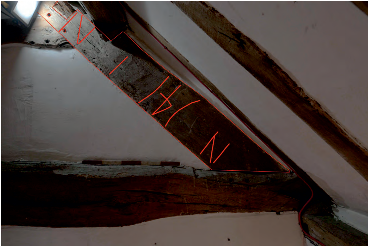
Truss No. 1 - detail of assembly marks and Baltic timber importers marks (probably North Prussian oak) on southern end of truss
