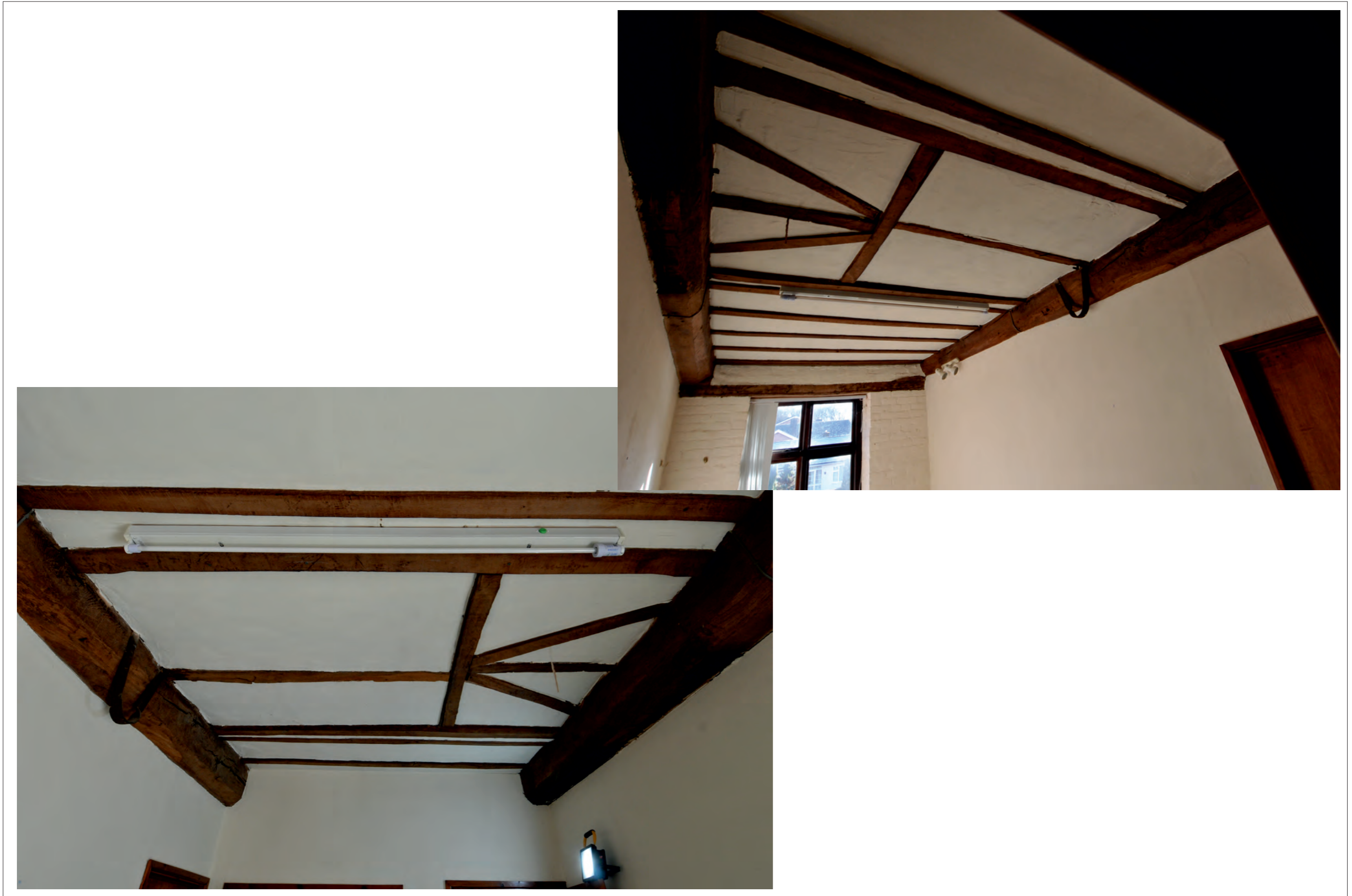
Figure 10: Probable former floor trap door location - note strap hanger
