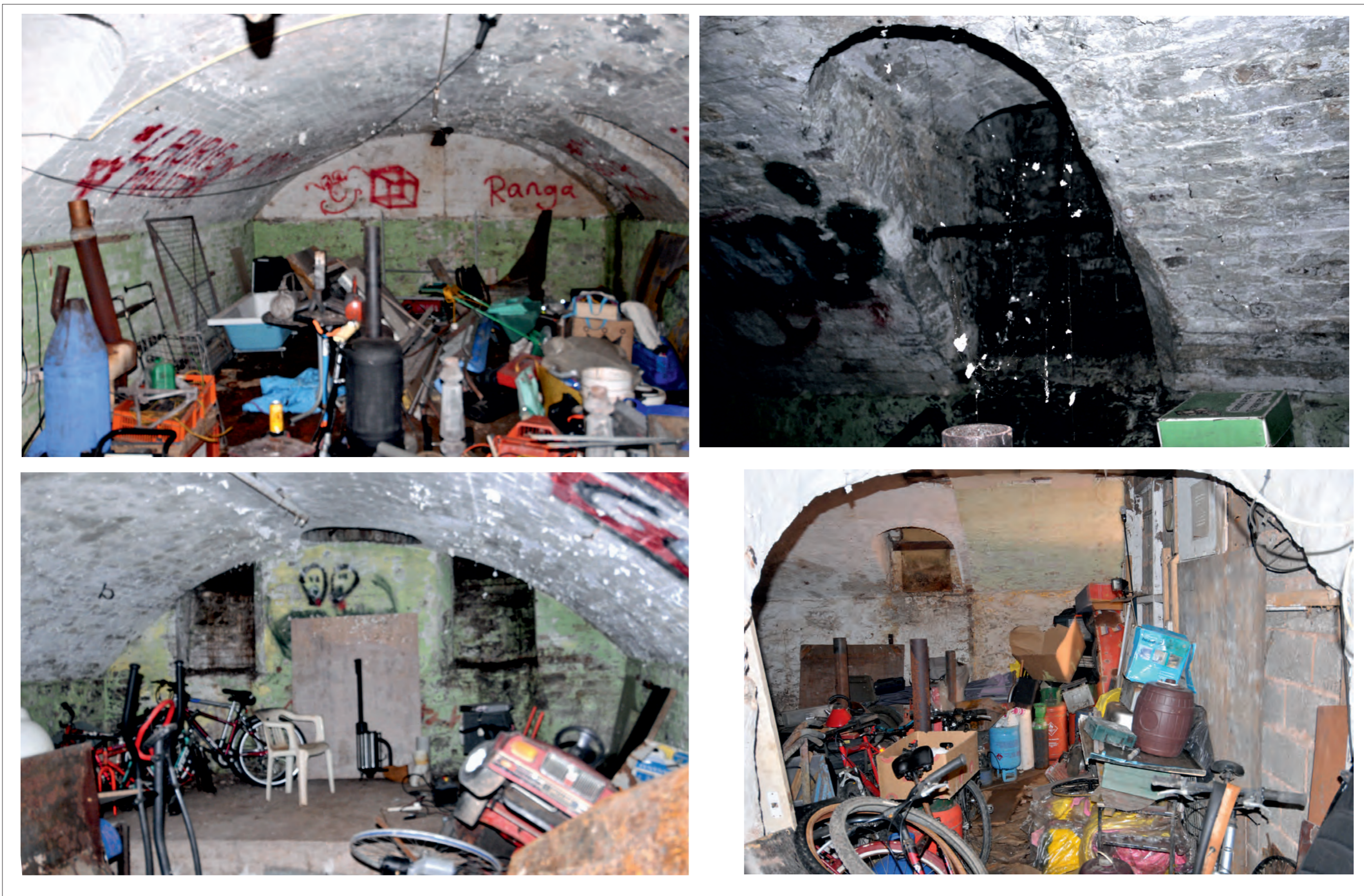
Figure 20: Basement area - Block 1
