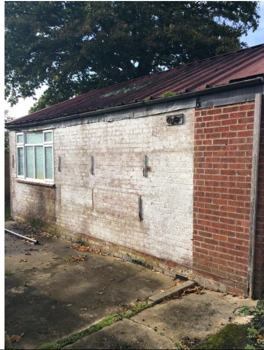
Left hand flank wall of garage
