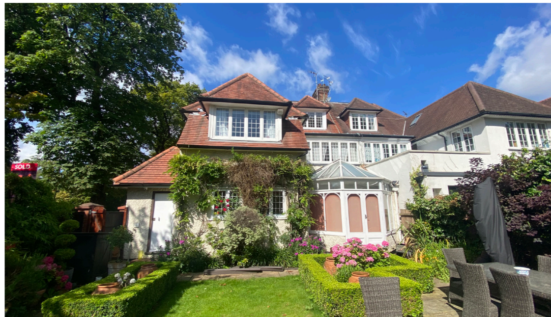
Fig 4. Existing Rear Elevation
