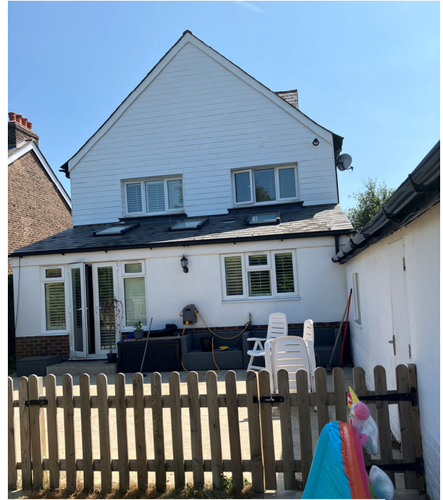
03 View of the rear of 208 Whyke Road
