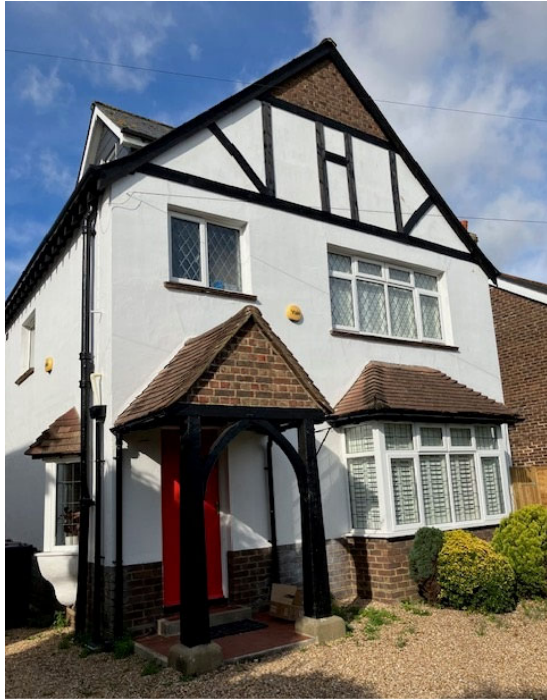
02 View of the front of 208 Whyke Road
