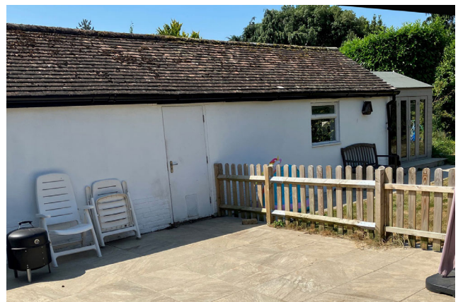
05 View of the end of the outbuilding and
