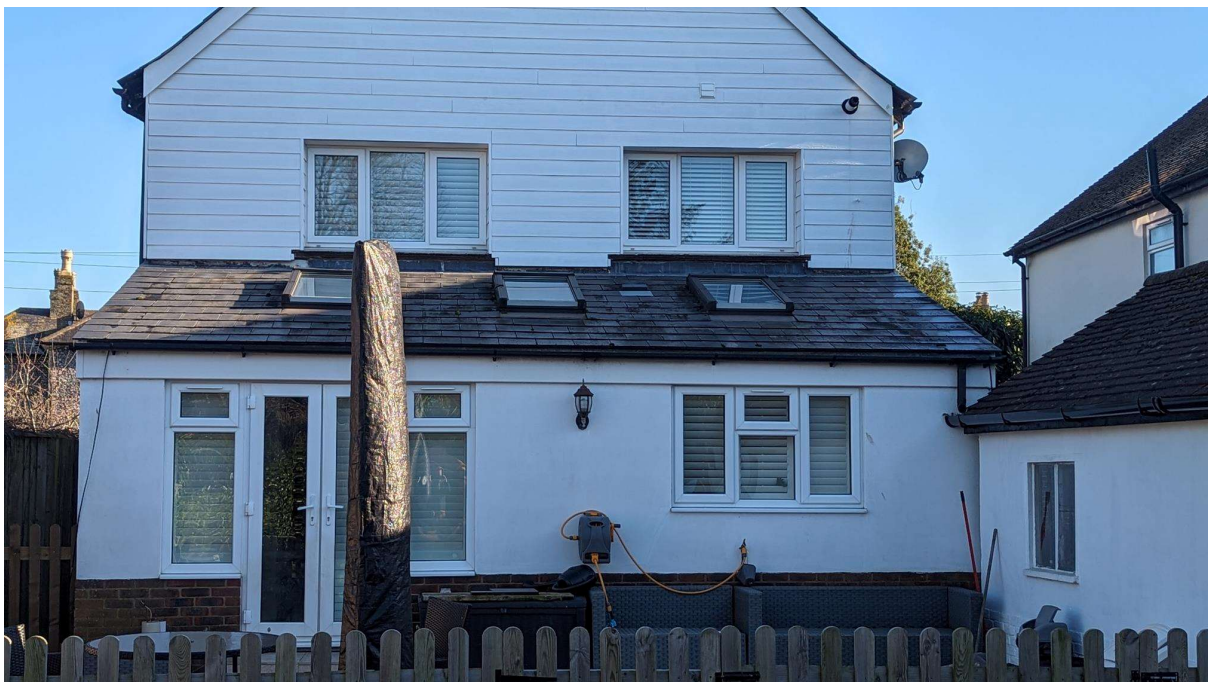
Photo 2 – View of the dwelling from the rear (west).
