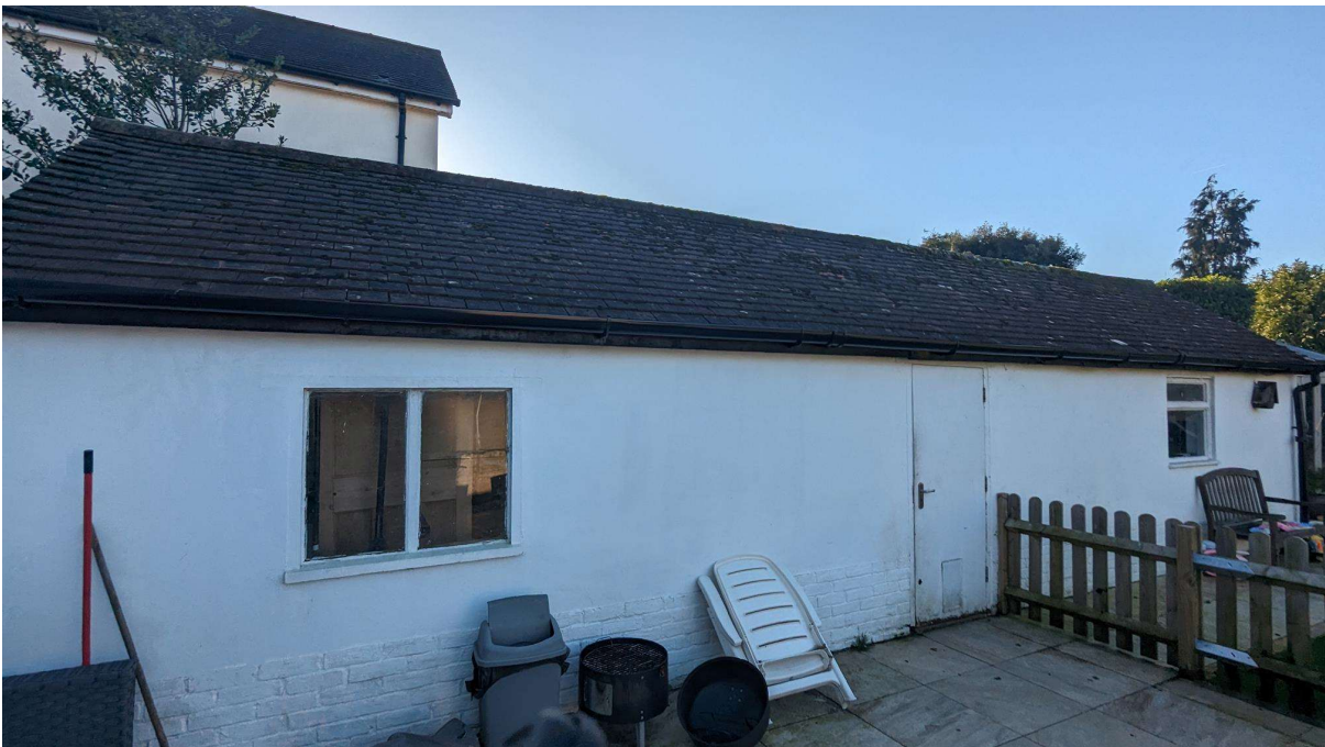
Photo 4 – View of the garage from the side (north).
