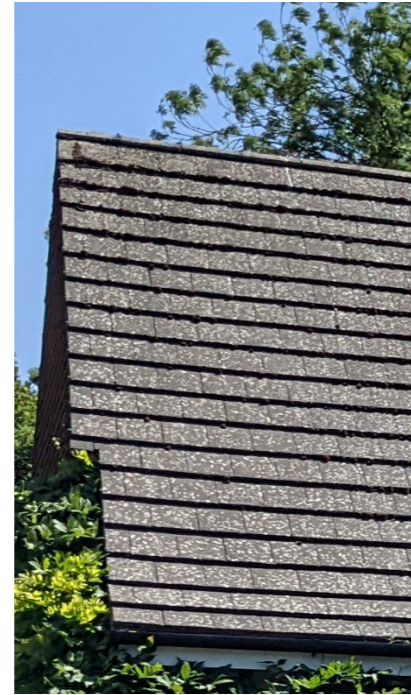
EXISTING ROOF Tiles
