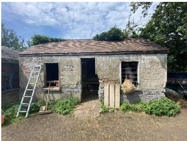
South face of B1
