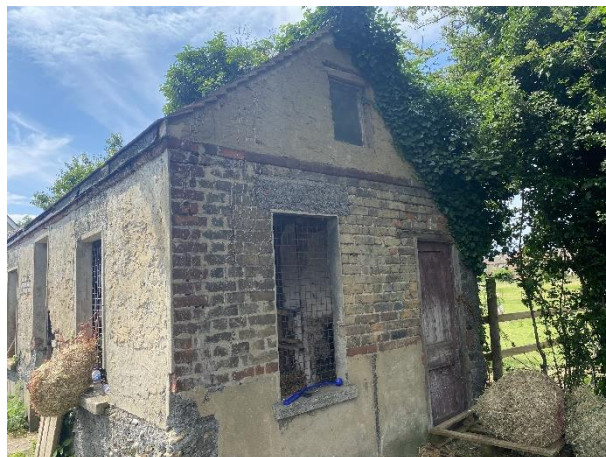
East face of B1
