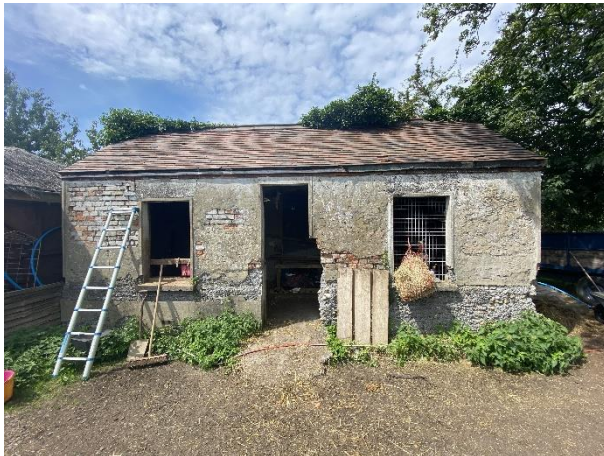
South face of B1
