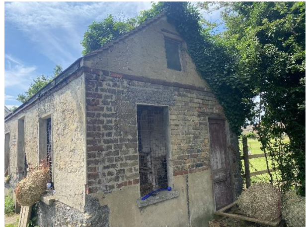
East face of B1
