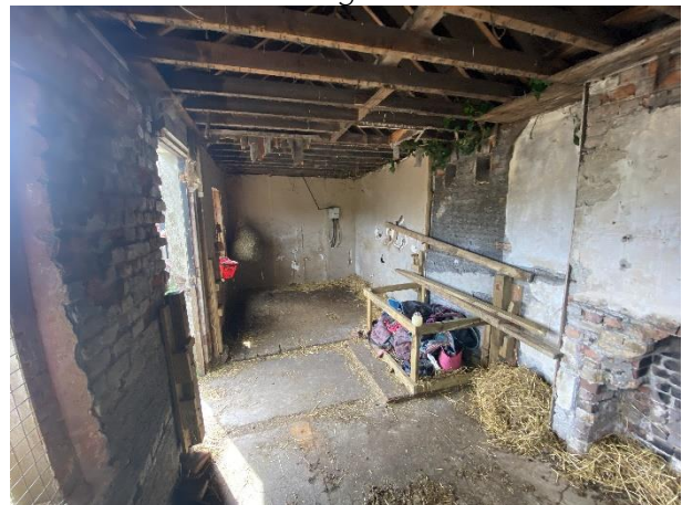
Interior. Fireplace and chimney stack pictured left.
