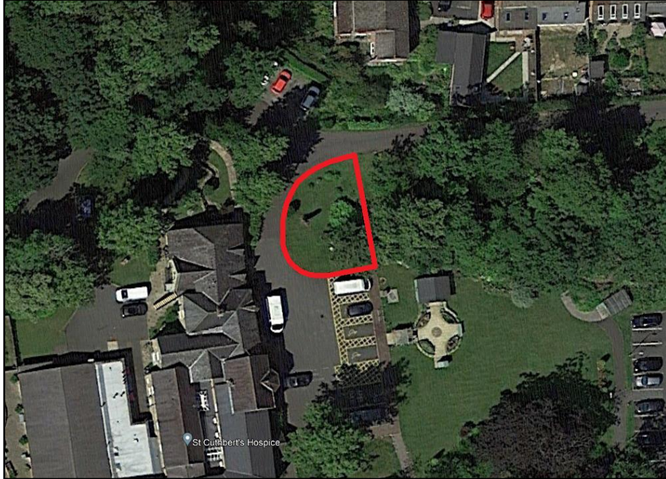
Figure 1 - The location of the proposed parking bays are indicated by the red line in the above image.
