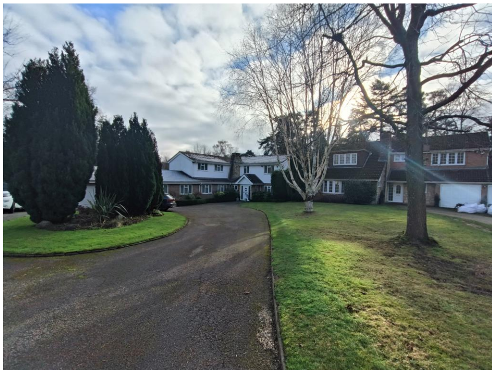
View of No.3 with double storey extension
