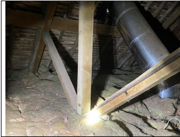
Photo 5 Loft floor section D dust-covered
