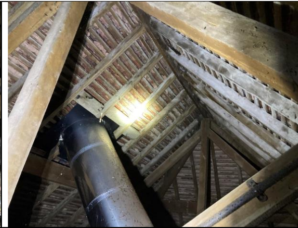
Photo 6 Section D unlined roof
