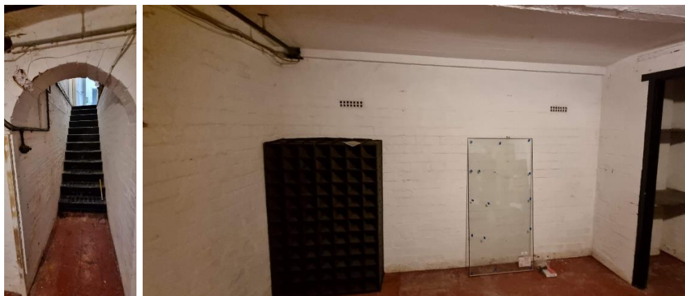
Images of existing basement and staircase.
