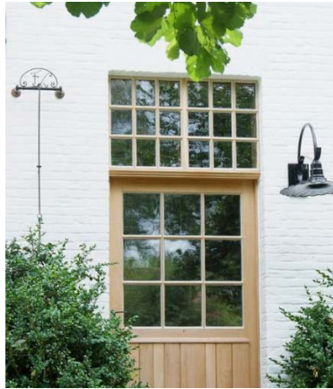
Painted Main Brick (Farrow & Ball 'Pointing')
