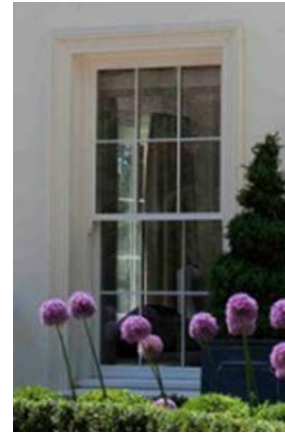
White Painted Sash Windows & Window Surround
