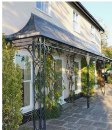
Standing Seam Lead porch with wrought iron posts
