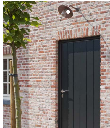
Side Extension Brickwork
