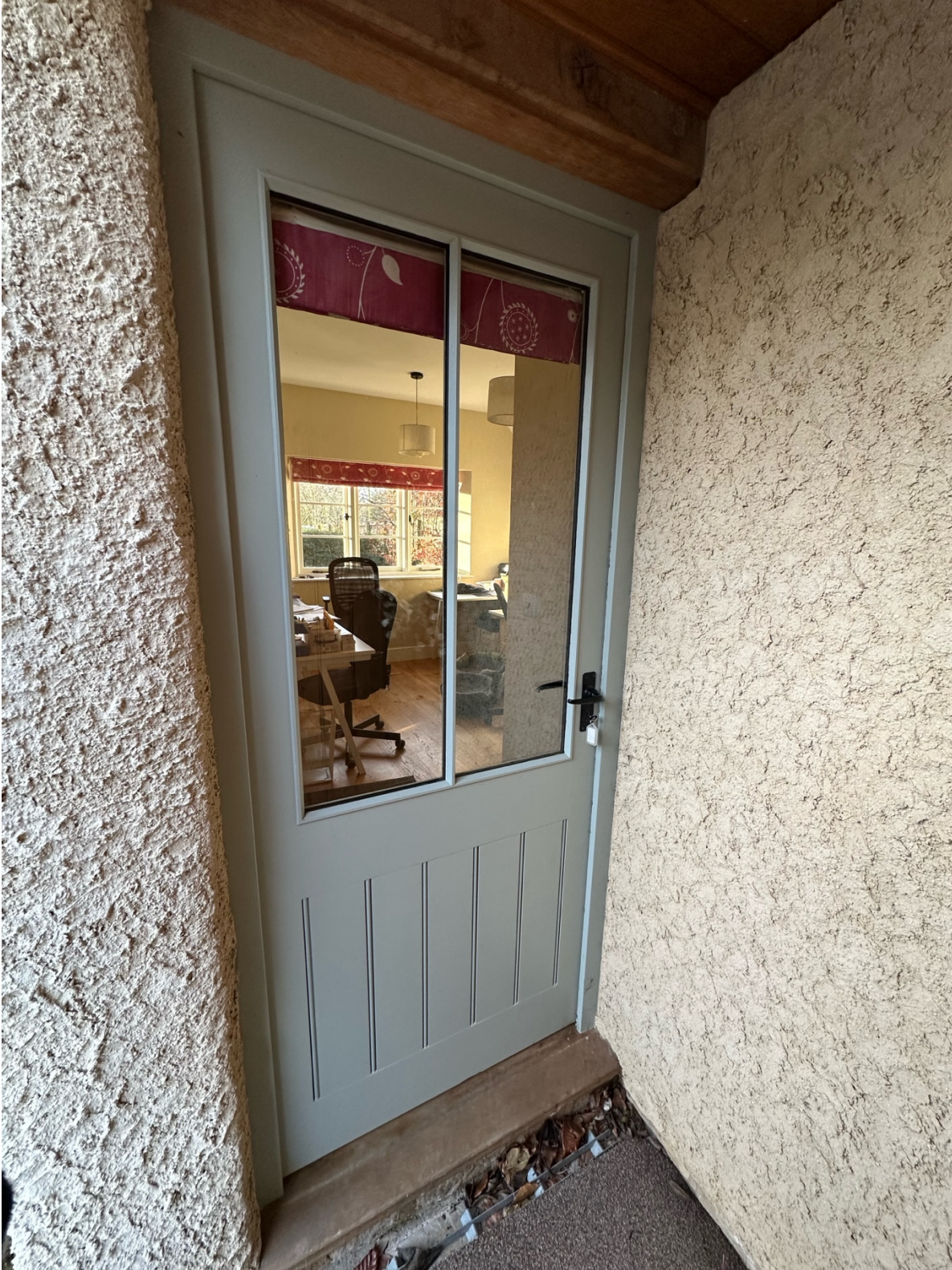
Existing door that will be matched
