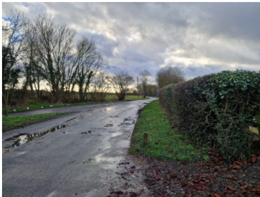
Figure 3: View N of Southern Access from edge of carriageway
