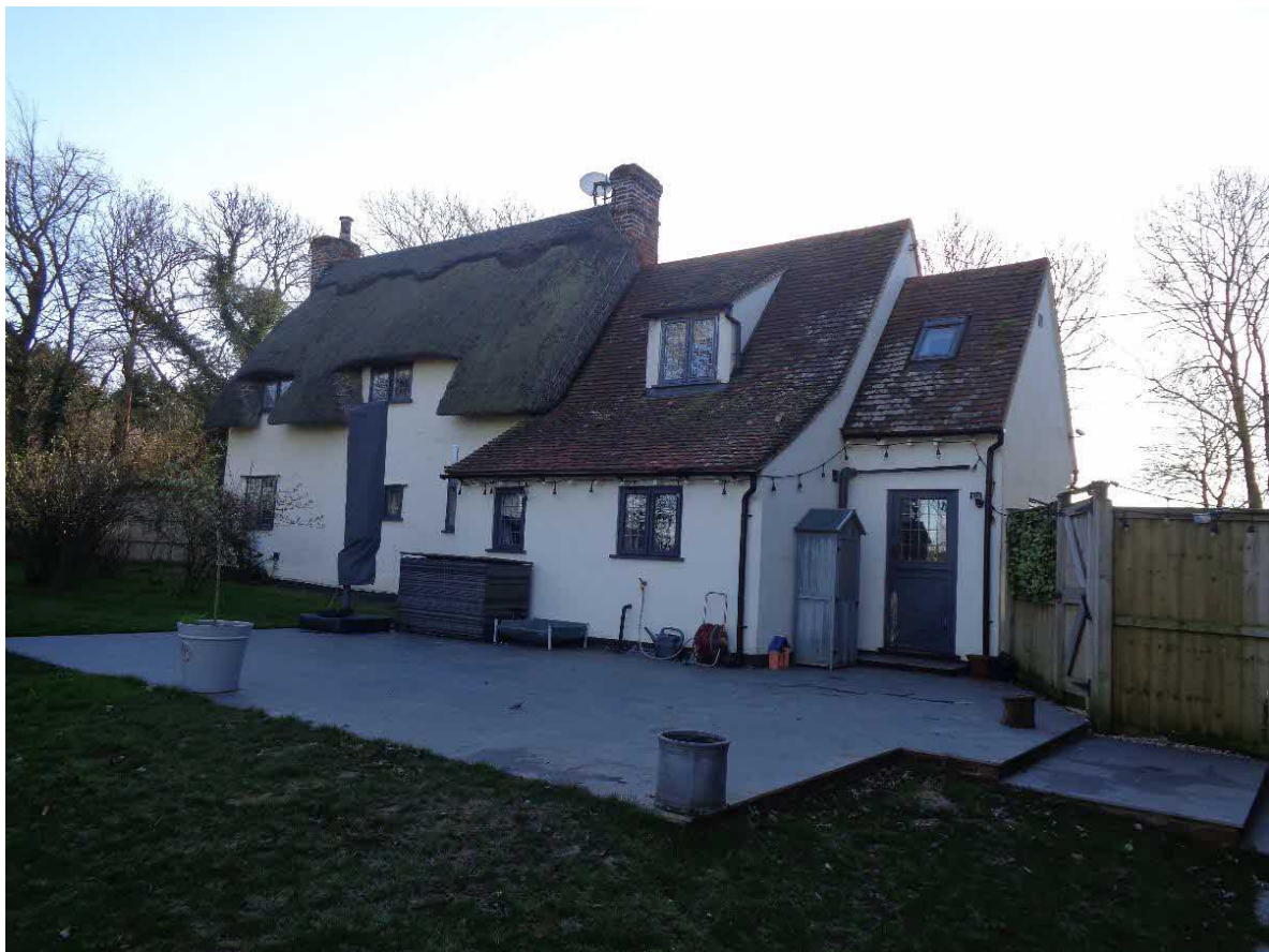
Rear elevation of the cottage
