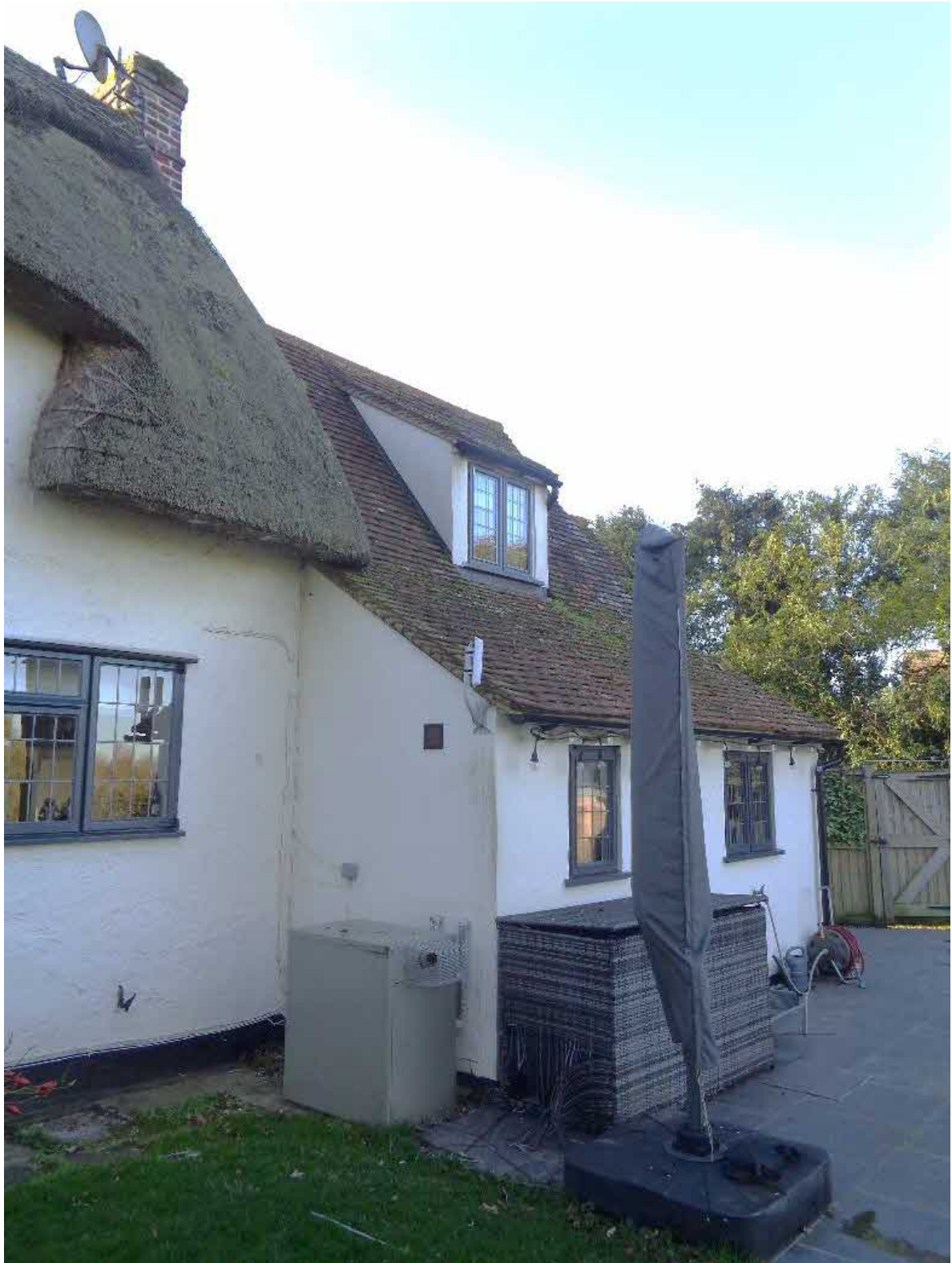
Existing rear extension
