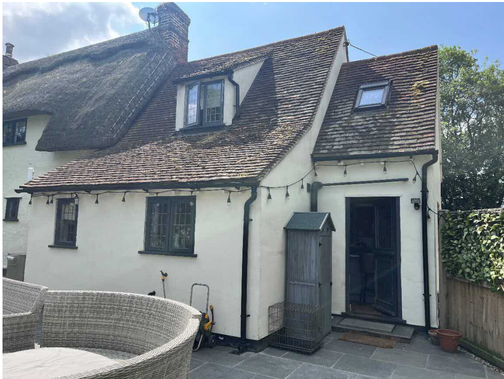
Rear of existing C21 addition
