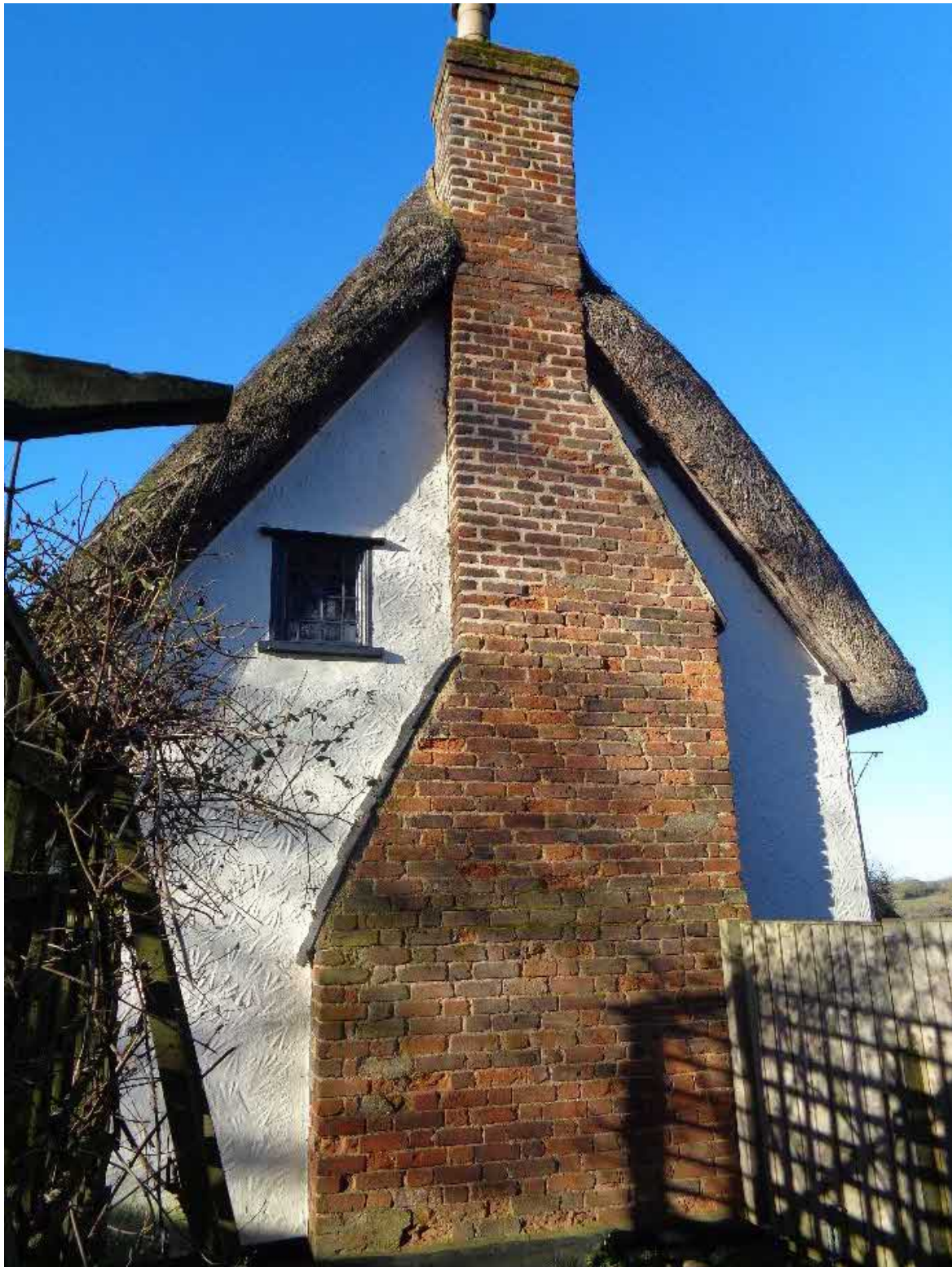
Eastern gable end
