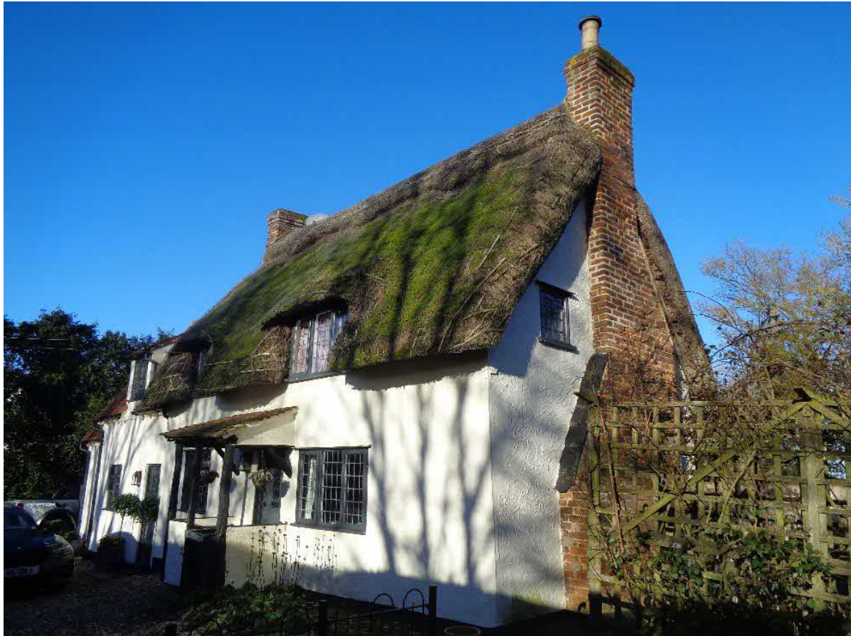
Southern elevation of application cottage
