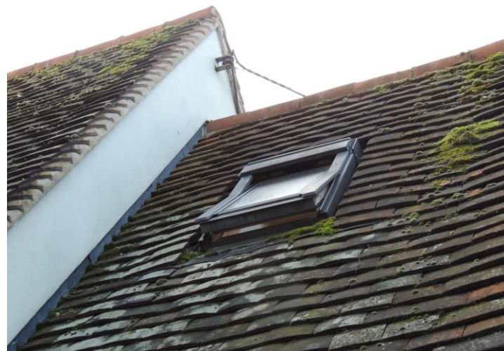
Photo 4: Showing tight seal to roof tiles and gable
