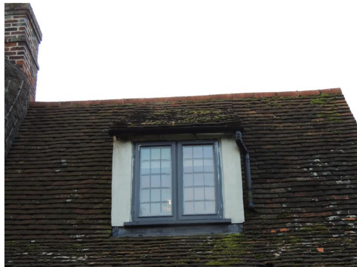
Photo 6: Showing tight seal to roof tiles
