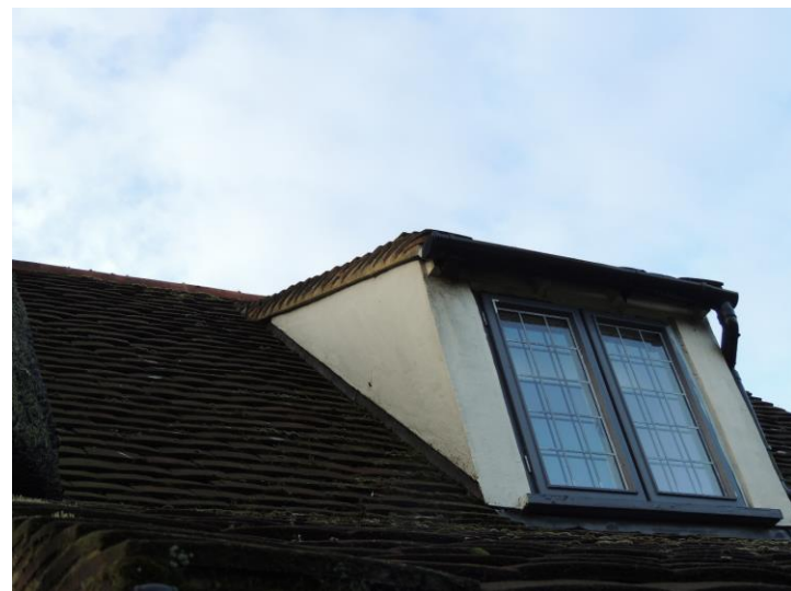
Photo 7: Showing tight seal to roof tiles and dormer
