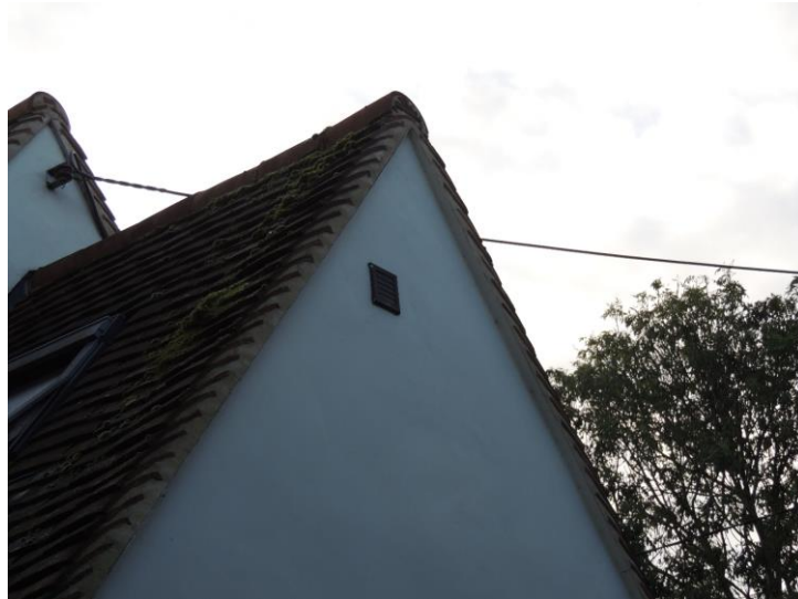
Photo 5: Showing tight seal to gable
