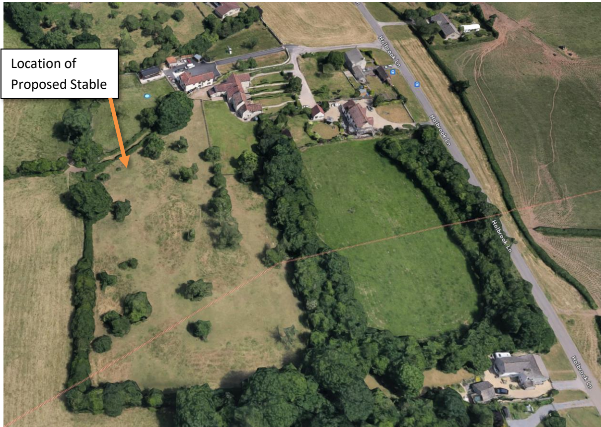
Figure 2 – Perspective Aerial View of the application site viewed in an easterly direction [source: Google Maps]
