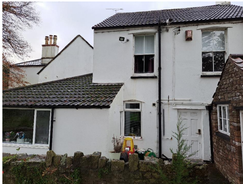
View of northern section of east elevation
