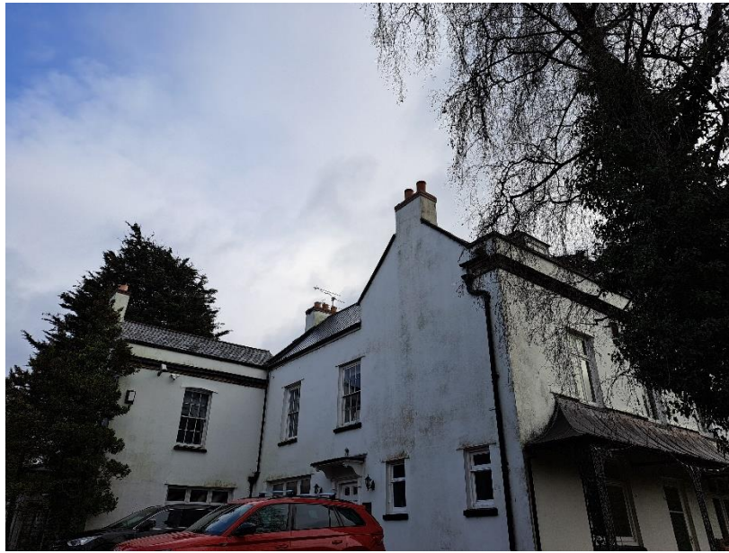
View of western section of north elevation
