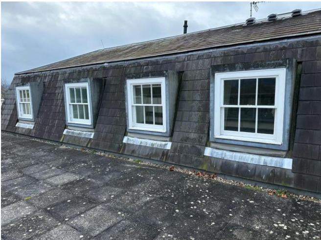
View of terrace including windows 1 to 4
