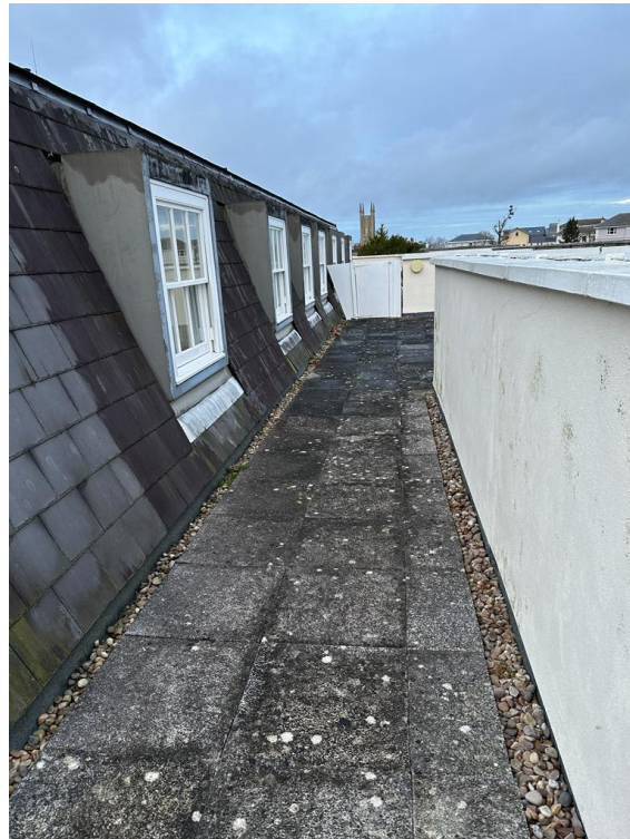
View of terrace including windows 1 to 4
