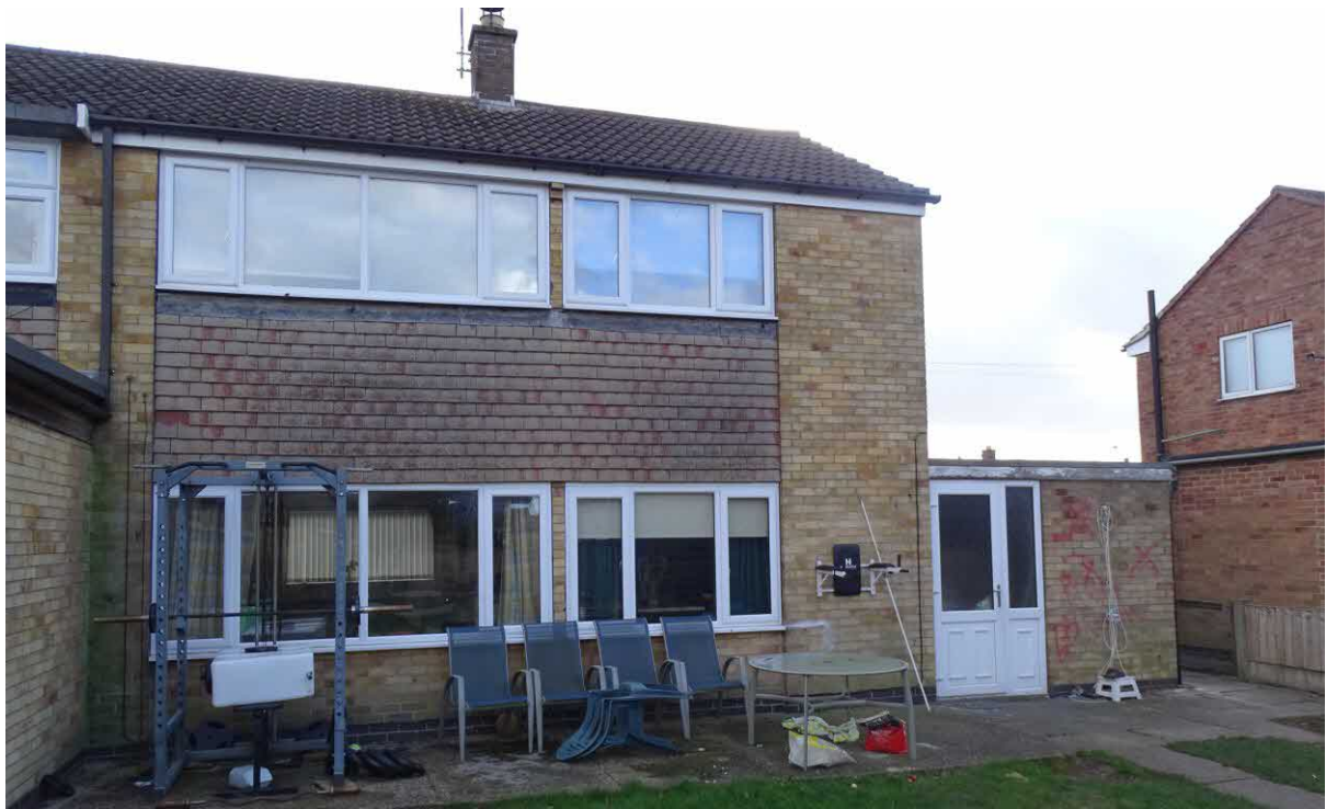
Image 3 – Rear North facing elevation of the property
