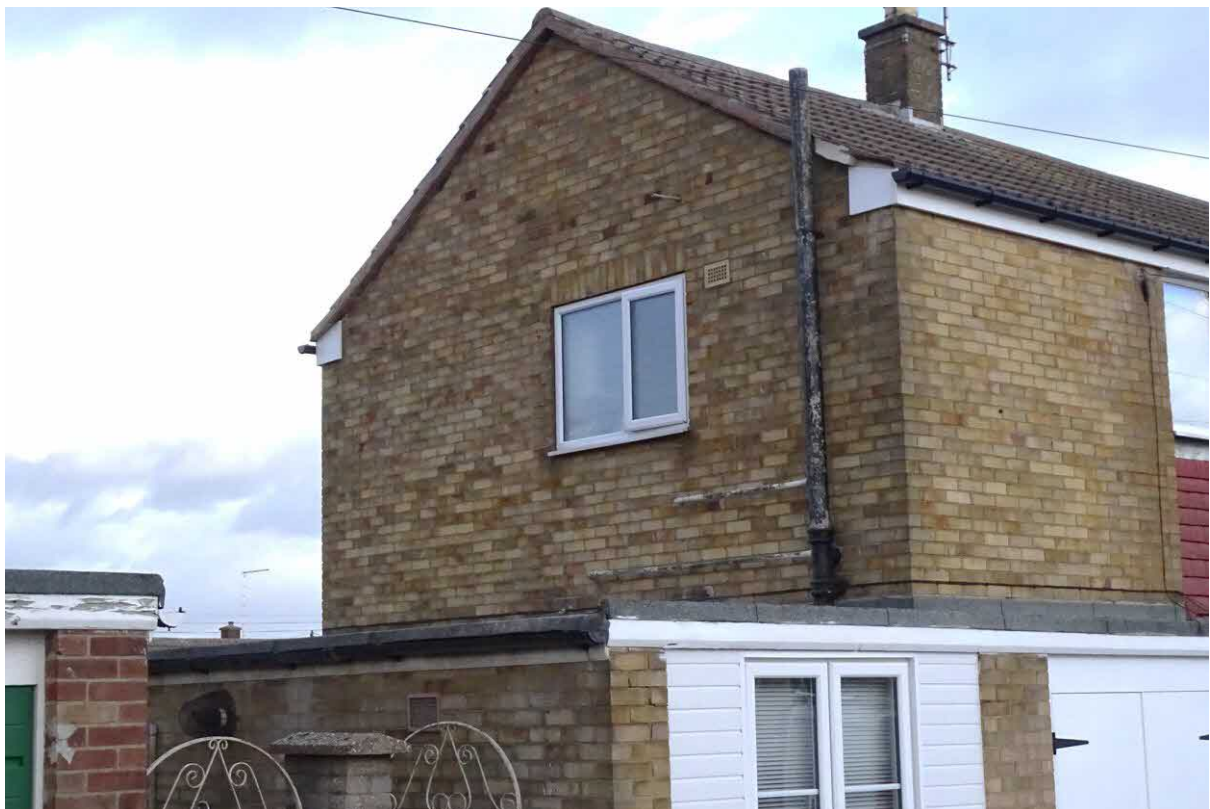
Image 2 – West gable elevation of the property
