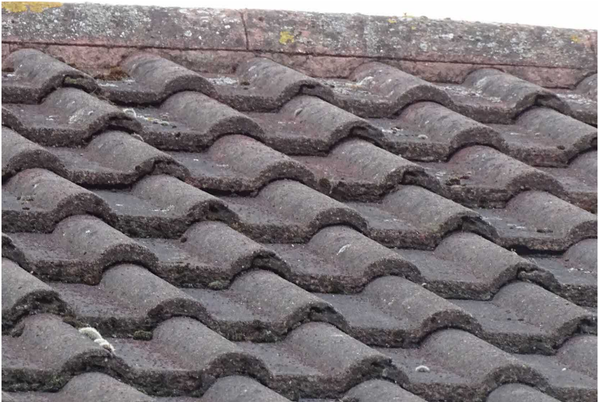
Image 5 – Close view of main upper roof coverings to demonstrate condition
