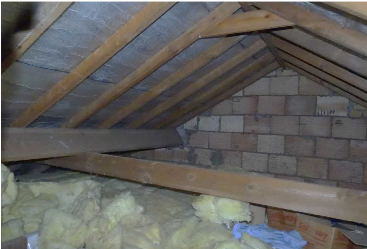
Image 6 – Internal view from within the main roof void spaces of the property
