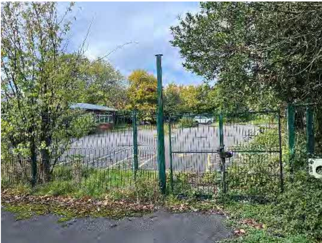
Plate 8. View from the north-west of the study site, westwards across the former car park
