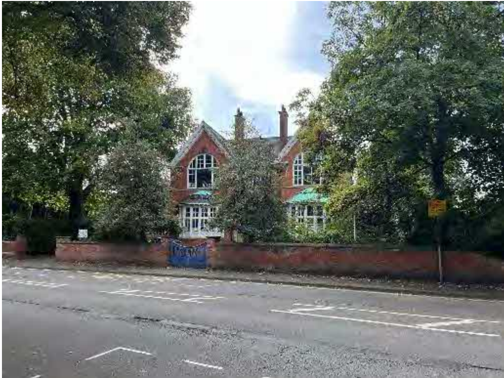
Plate 1. Frontage of the former Lilley & Stone School building (Block 2) Grade II Listed building, facing south-east across London Road, showing the northern boundary of the study site
