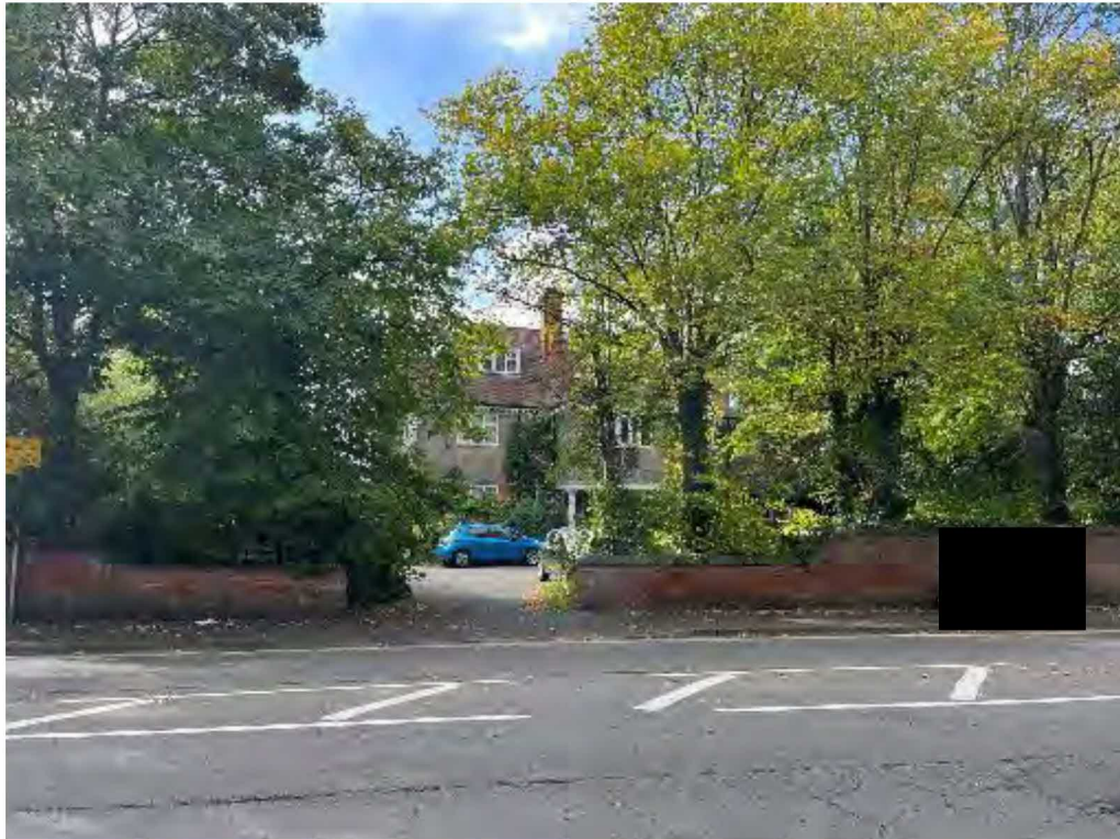
Plate 4. View of the frontage of the former headteacher's house (Block 1), facing south-west across London Road
