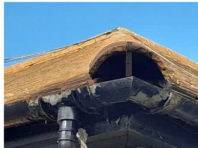
Southern elevation of B12 with slipped hanging tiles
