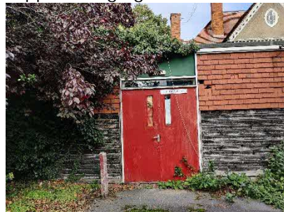
Southern elevation of B12 with slipped hanging tiles
