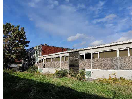
Figure 12 Example of G2 habitat adjacent to building 6.
