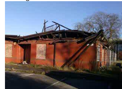
Eastern elevation of B6 following fire damage
