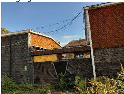
Cracks in wooden slats and hole in hanging tiles of B5
