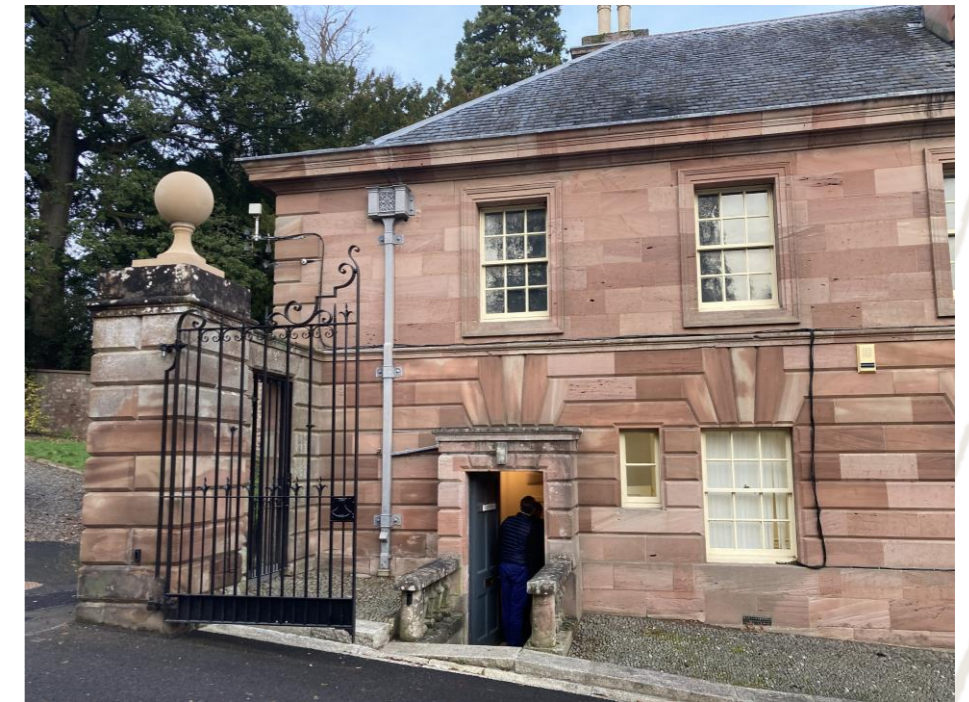
Fig. 14 External entranceway to west elevation of Estate Offices
