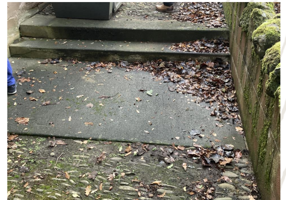
Fig. 15 External steps to gable entrance
