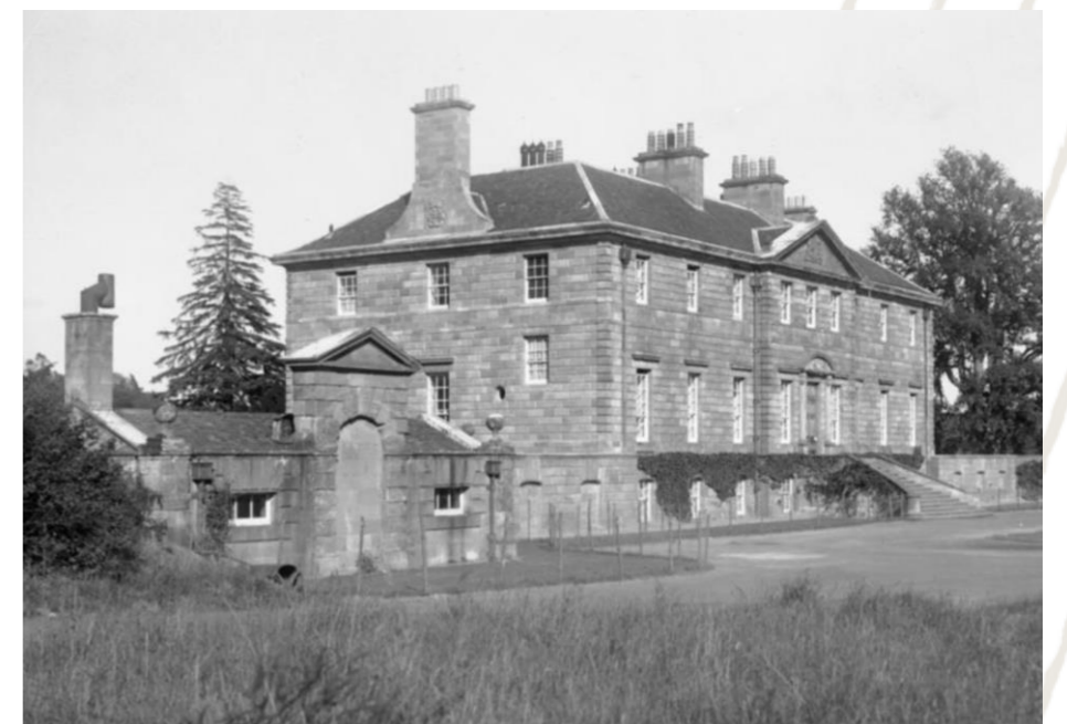
Fig. 19 Image illustrating completed scheme by Ian Lindsay, 1954.
