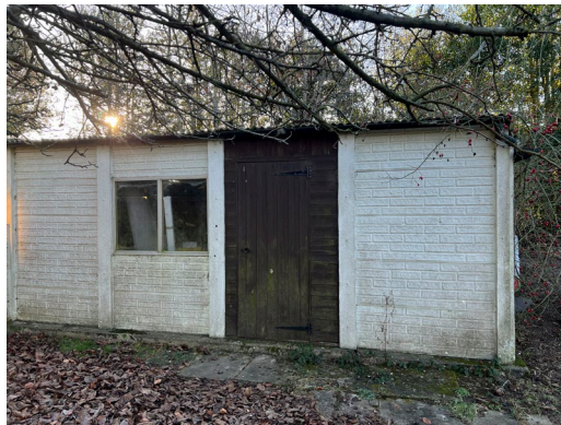
South View of Garage / Store
