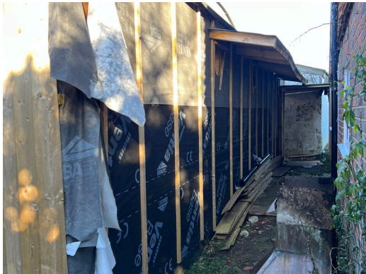
North West View of Timber Frame Structure
