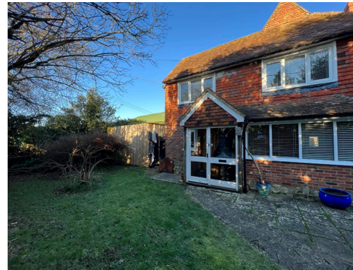
North West View of Butlers Farmhouse and Adjacent Timber Frame Structure
