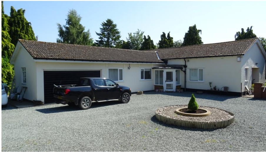
Figure 4.4. South side of bungalow and gravel driveway
