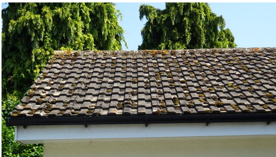
Figure 4.8. Well-set roof tiles
