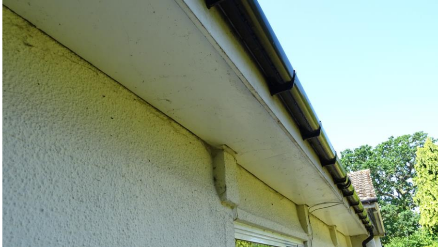
Figure 4.9. Well-sealed soffits
