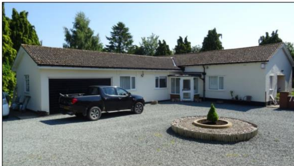
Existing front elevation of single storey property below
