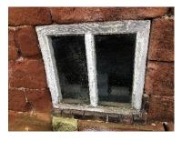
With regards to the window design then the proposal is that the current design is retained, with no cross bar. Unfortunately due to their age, wood worm infestation and general rot the current windows cannot not be repaired, however by retaining the existing design the original character/look of the barn will be retained.
