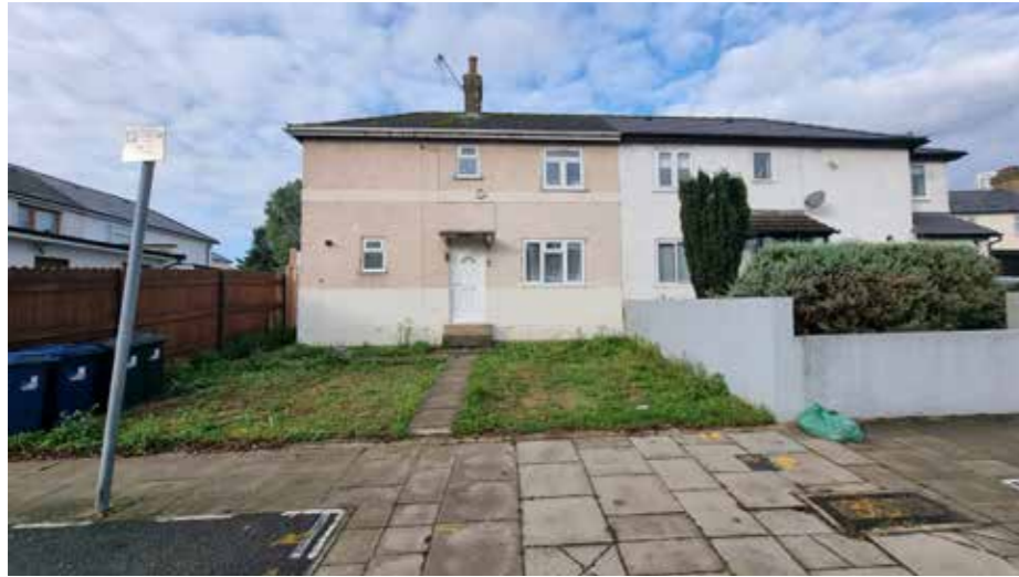
Front elevation onto St. Andrews Road(East facing)
