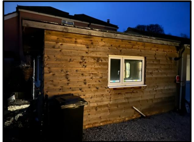
Figure 8 Side elevation of rear to garage/annex
