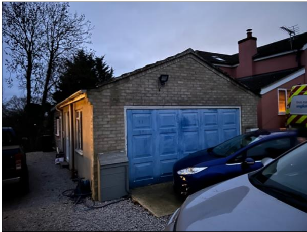
Figure 7 front view of existing garage/annex
