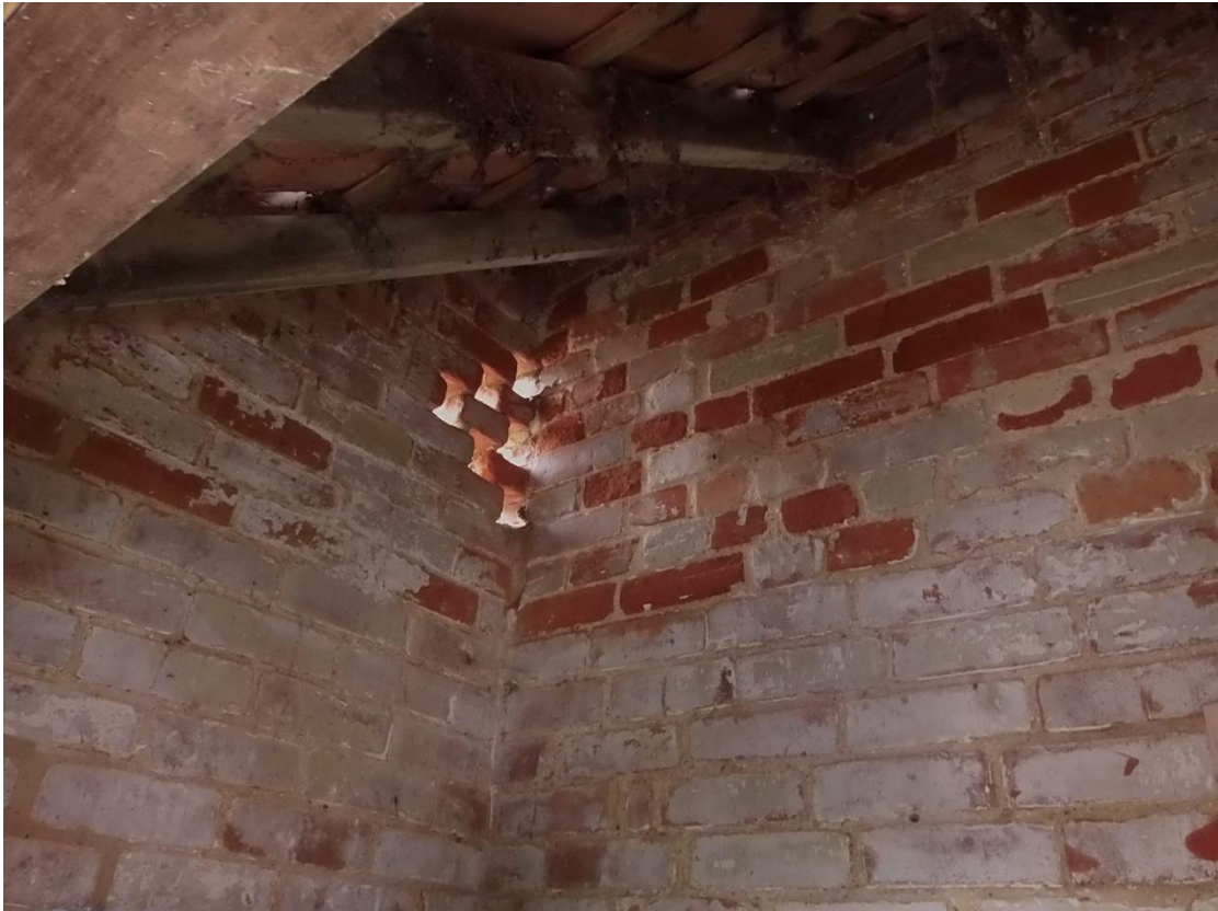
Photo 10 , internal view of building two, looking northeast.
