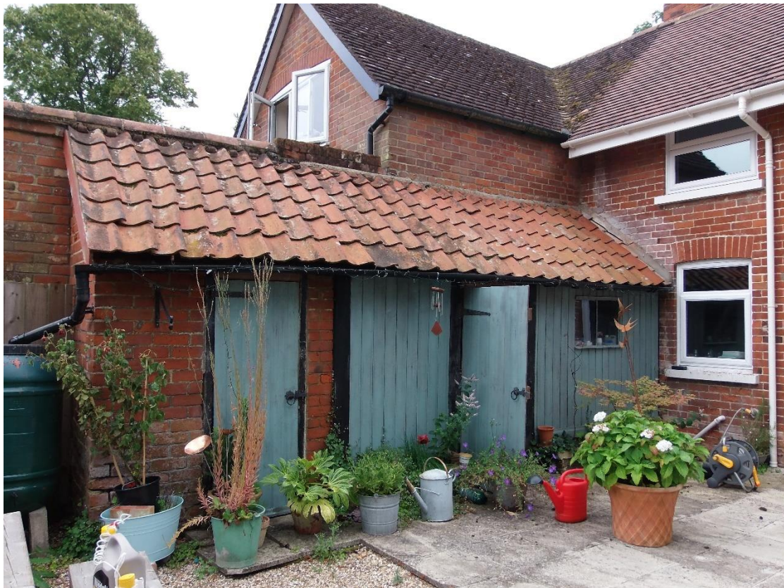
Photo 9 , north and west aspects of building two.
