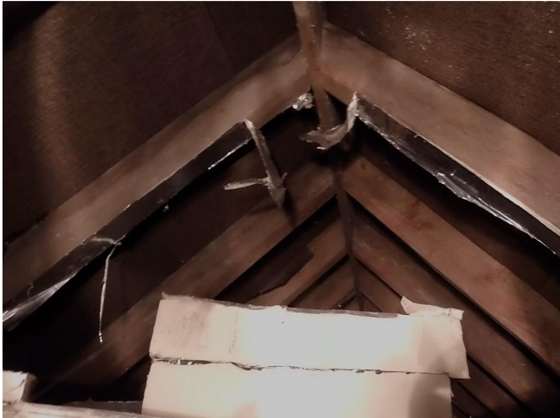
Photo 7 , internal view of building one, looking south.
