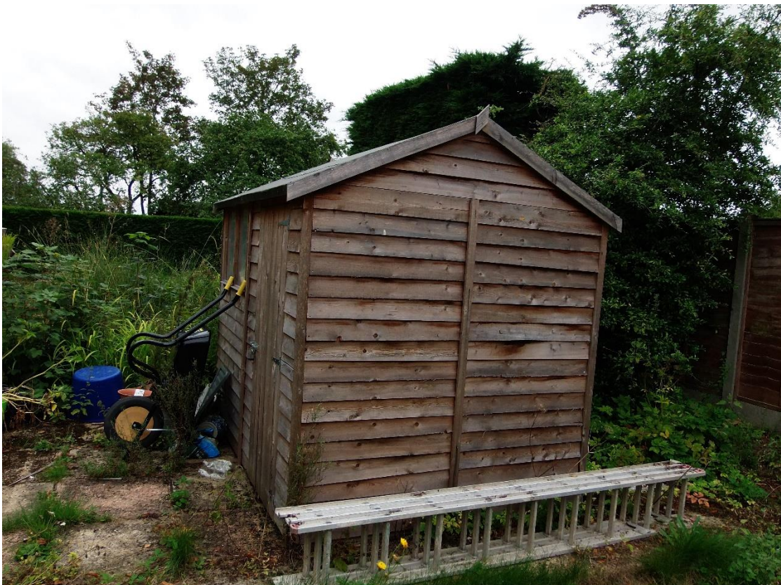
Photo 12 , south and west aspects of building four.
