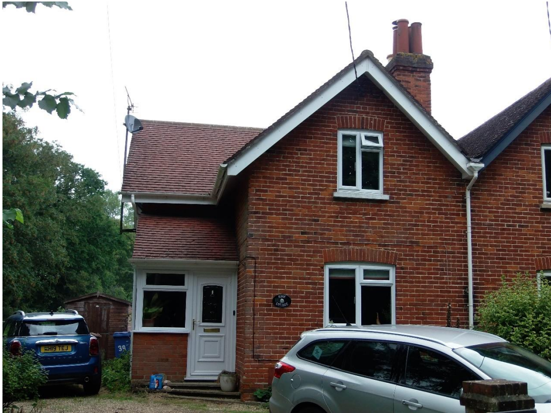
Photo 7 , south aspect of building one, looking north.
