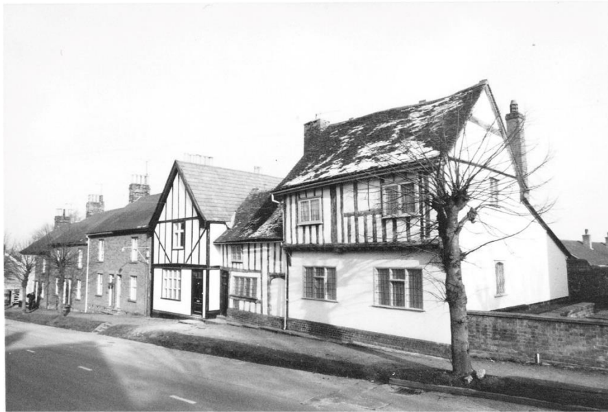
Fig 4. Both 57 and Yaxley Cottage were subsequently renovated.
