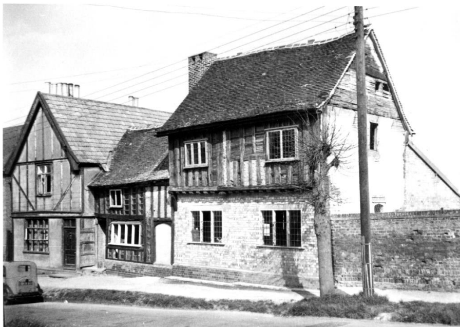
Fig 3. By the early 20th century, the pantile roof covering has been replaced with slates, the render removed and replaced with applied 'sham' timber framing to a jettied first floor and the two windows at ground floor replaced by one large window.
