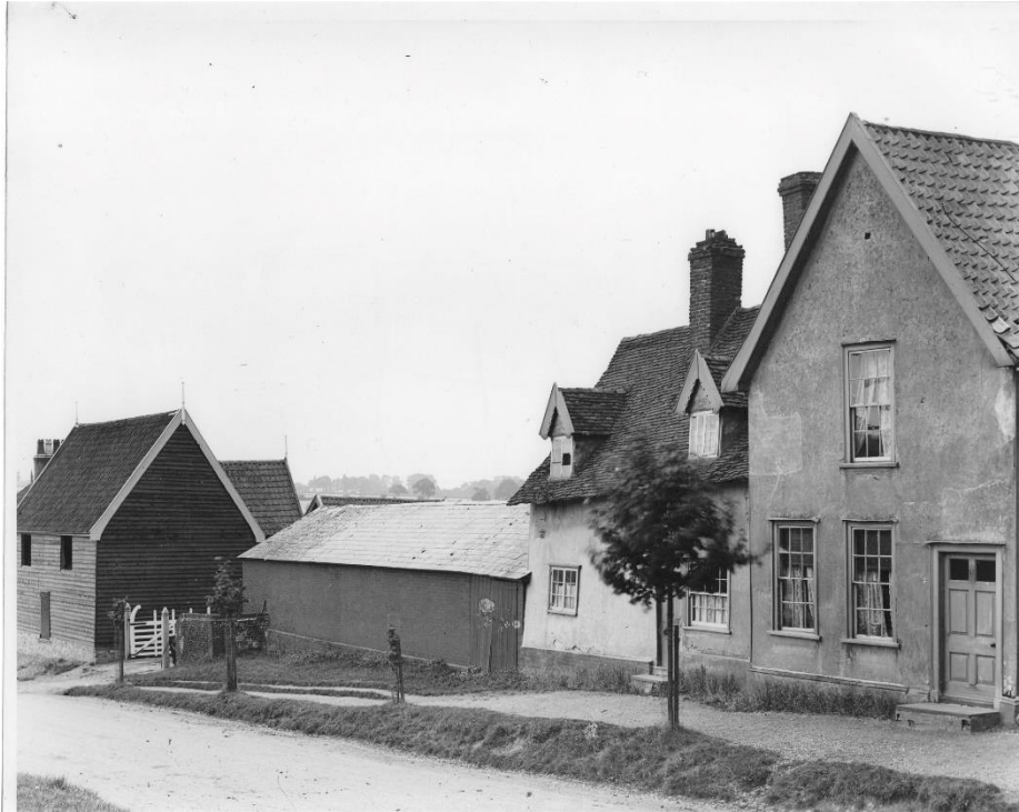
Fig 2. Early photographic evidence (Fig 2) shows the west elevation containing 3No sash windows, a uniform rendered appearance and a pantiled roof.
