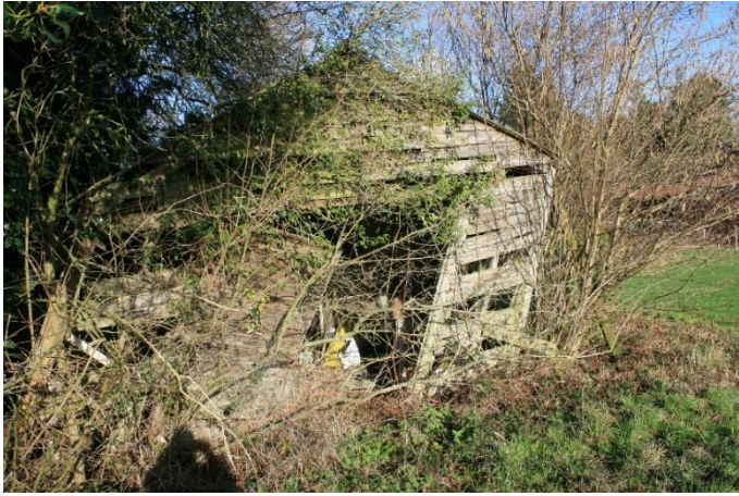
Photo 7: Southern elevation of 'Building 2'.
