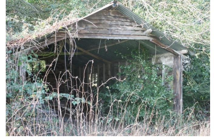
Photo 3: Eastern elevation of 'Building 3'.
