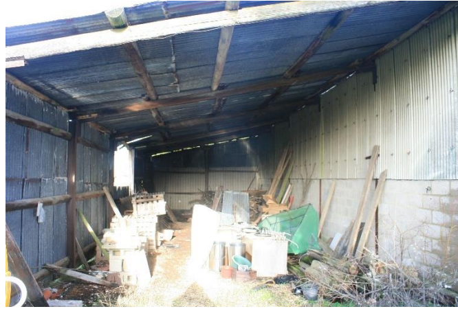
Photo 2: Internal area of 'Building 1'.
