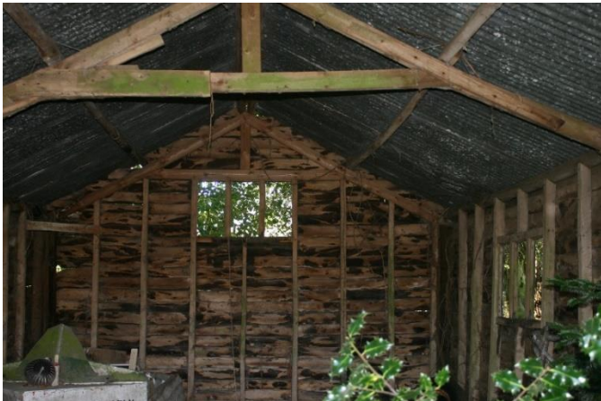
Photo 4: Internal area of 'Building 3'.
