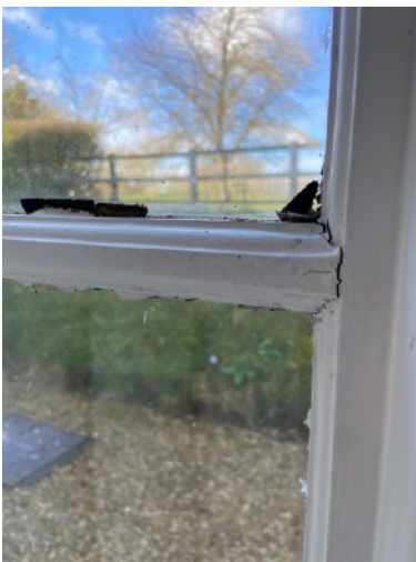
Existing French Door glazing bars- doors and side lights.
