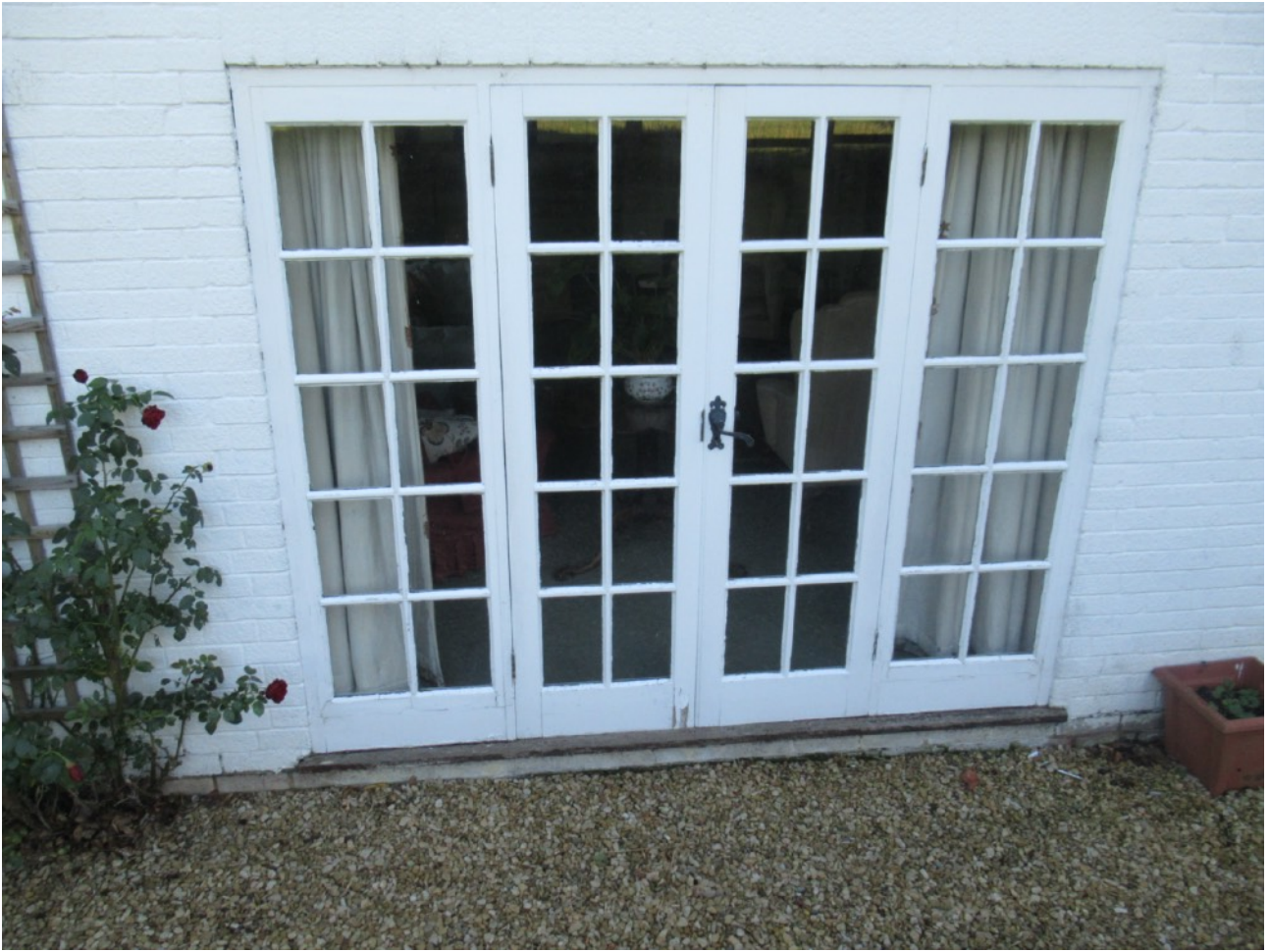
Existing French doors, with side lights.
