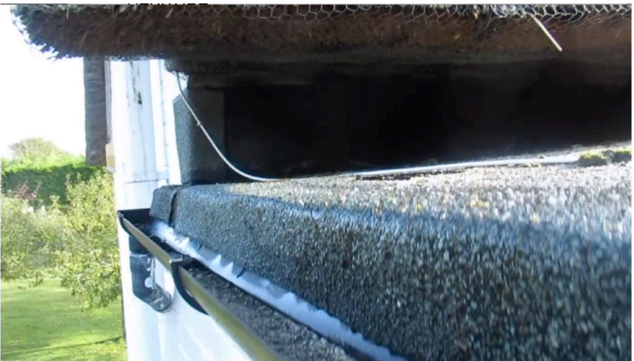
View across flat roof. Viewing from front to rear. Thatch to left slope sits on flat roof. Thatch to 1979 extension clear of flat roof.
