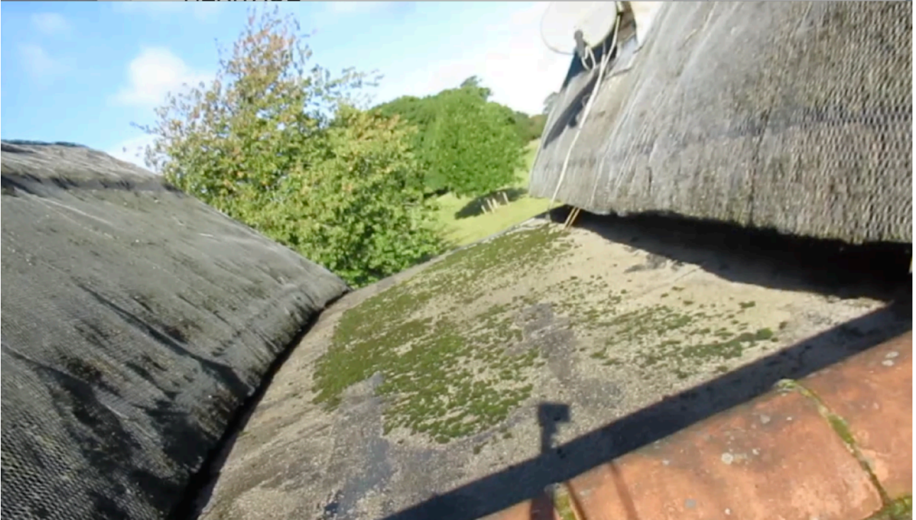
View across flat roof. Viewing from front to rear. Thatch to left slope sits on flat roof. Thatch to 1979 extension clear of flat roof.
