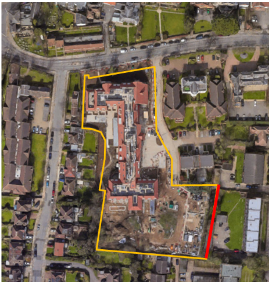
Figure 1.1. Aerial view of Barnet Grange Care Home, with the extent of its boundary in yellow and the wall in red
