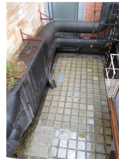
EXISTING GLASS BLOCK SKYLIGHT
