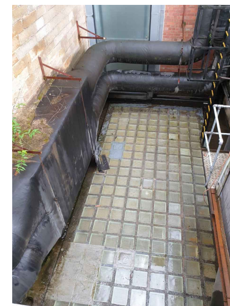
EXISTING GLASS BLOCK SKYLIGHT
