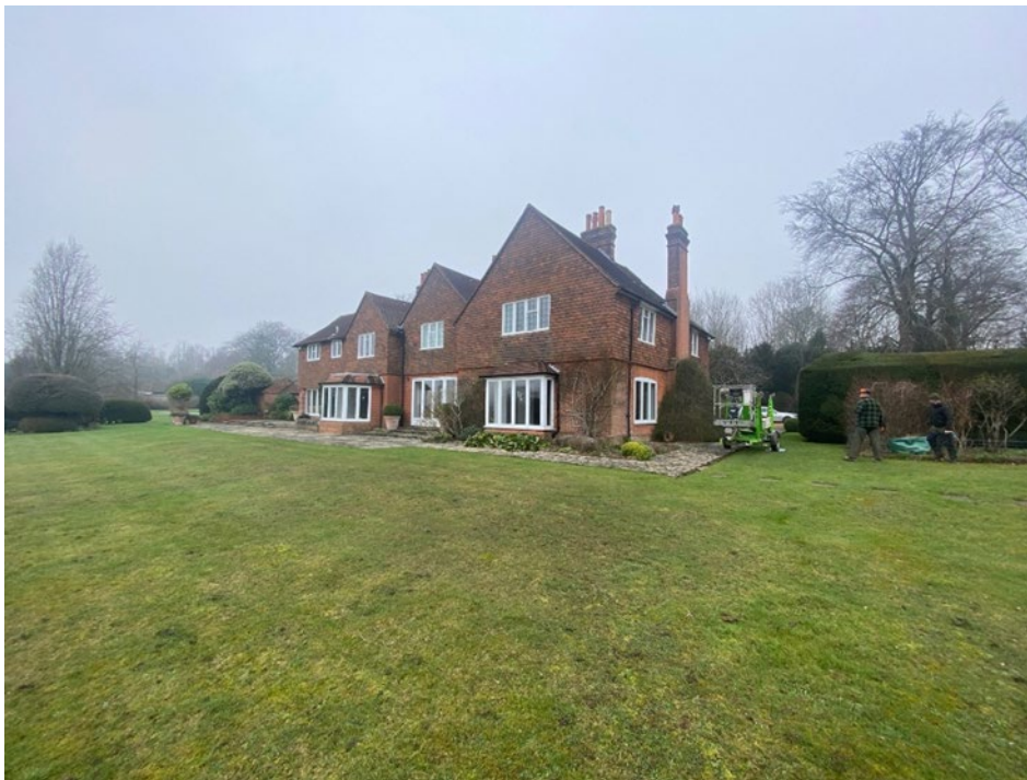
Rear and east side elevations: 2023
