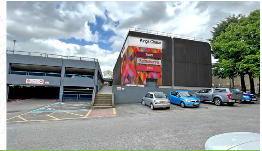
c. North Entrance: Facade and signage uplift to north entrance from existing multistorey and surface car parks
