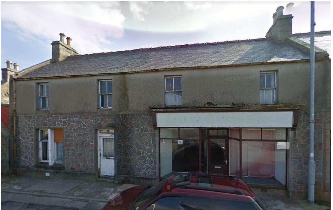
Above: Google Streetview image c.2011 showing historic windows & shopfront configuration. Intention shall be to replace the windows to match the sash & case configuration and format shown
