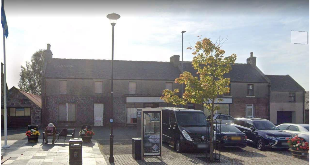
Above: Google Streetview image c.2021 showing window openings boarded up & missing chimney cans.
