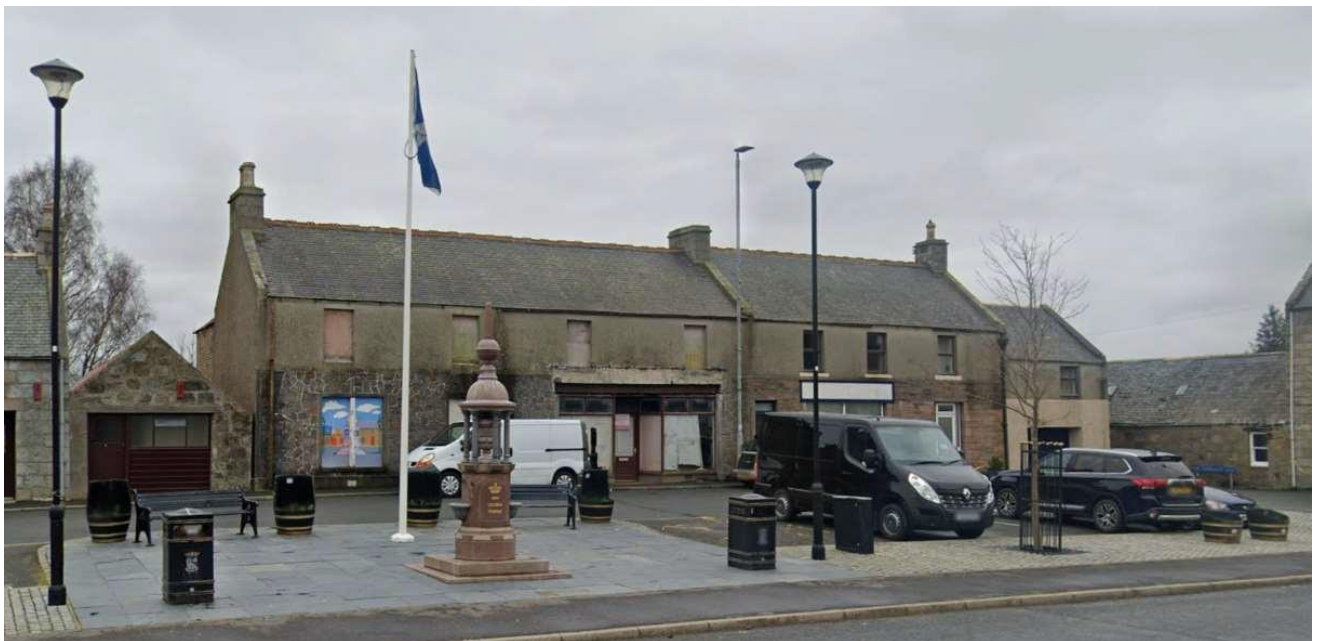
Above: Google Streetview image c.2023 showing window openings boarded up & missing chimney cans.
