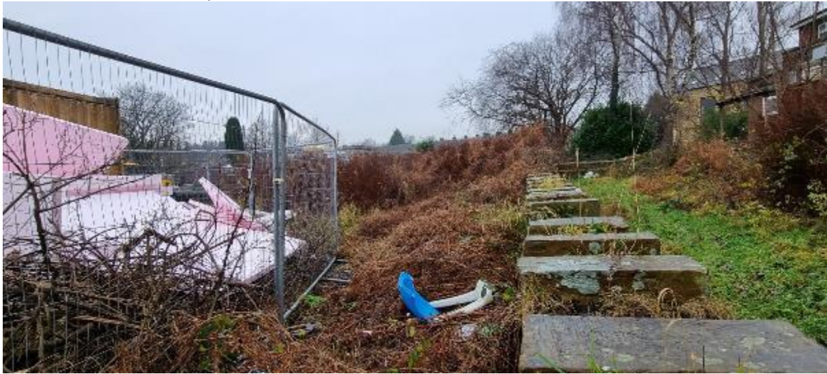
The far western boundary into the construction site (construction material to be removed)
