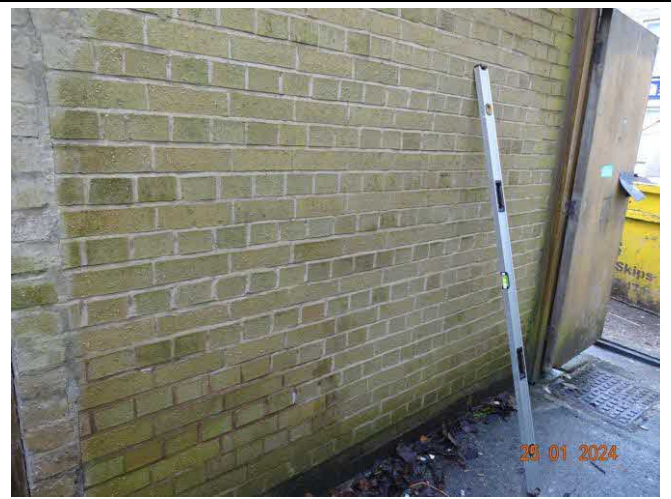
Photo 2 – Left hand side wall – front solid wall area.
