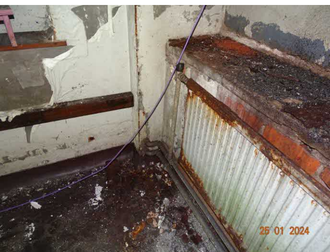
Photo 11 – Office structure interior showing rear retaining wall lower plinth and radiator.
