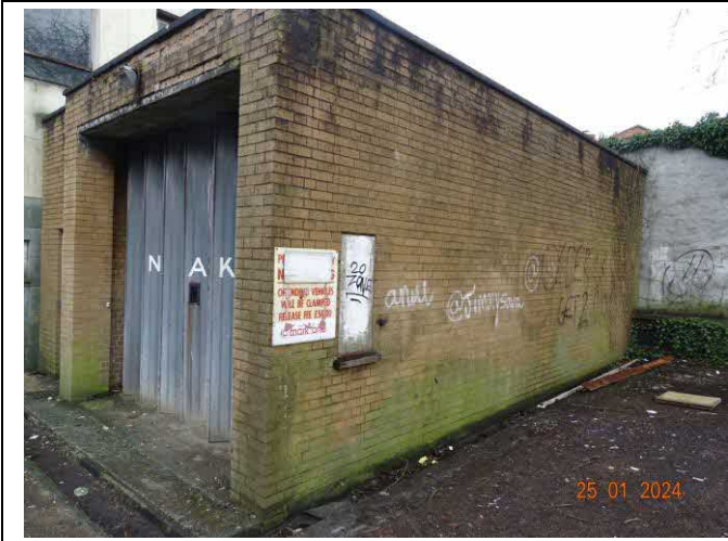
Photo 1 – Right hand side wall with front pier.
