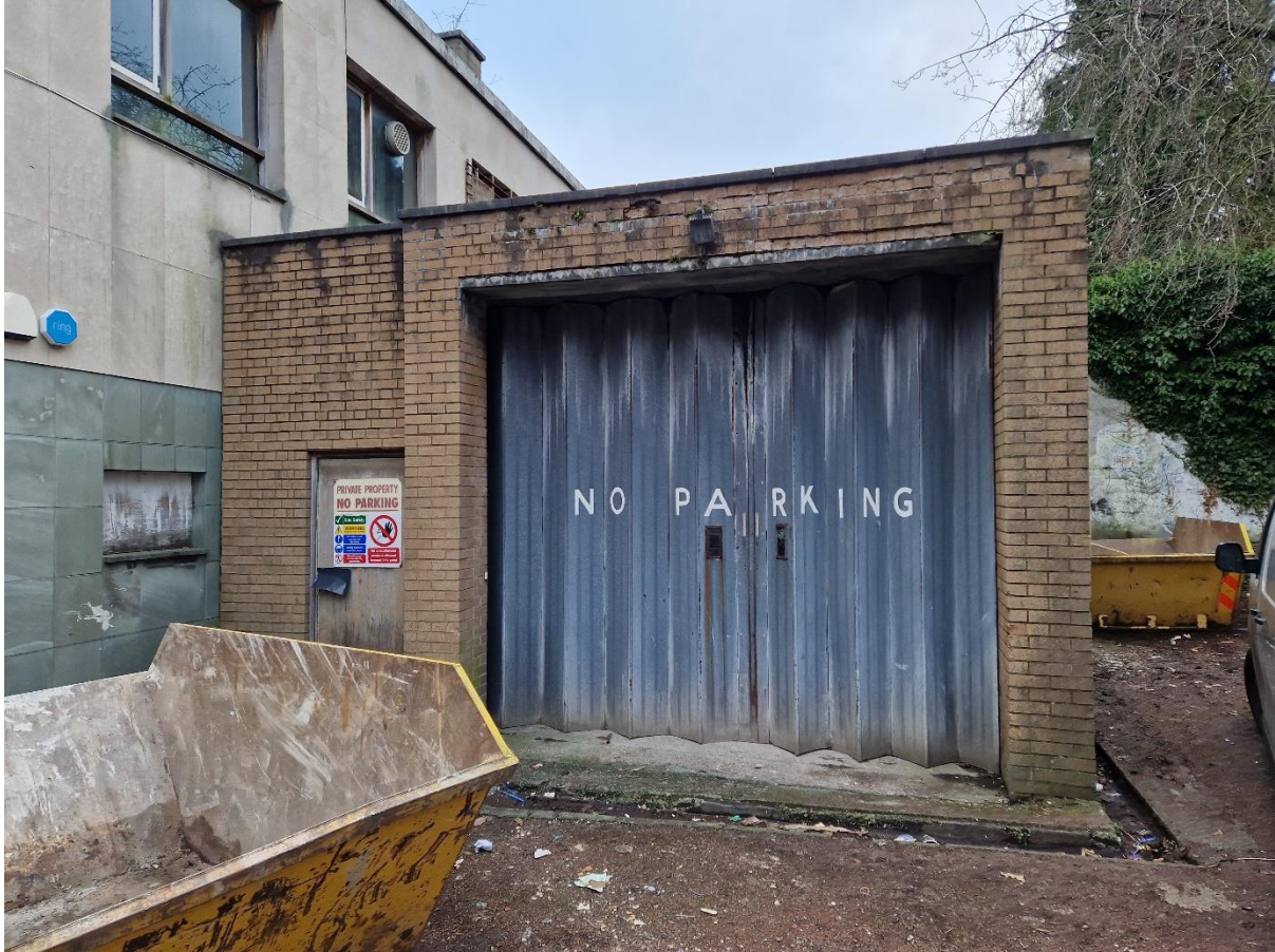
Figure 1: Front elevation of garage
